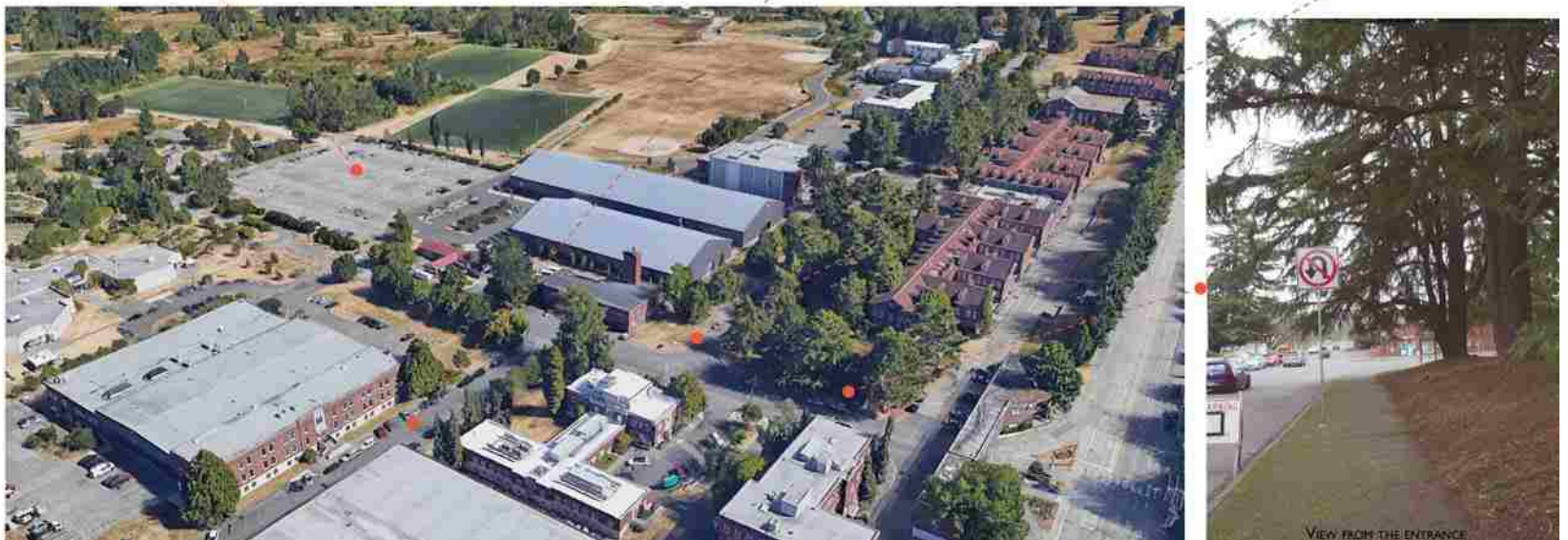
Figure 46. Aerial picture Source: Google Map
