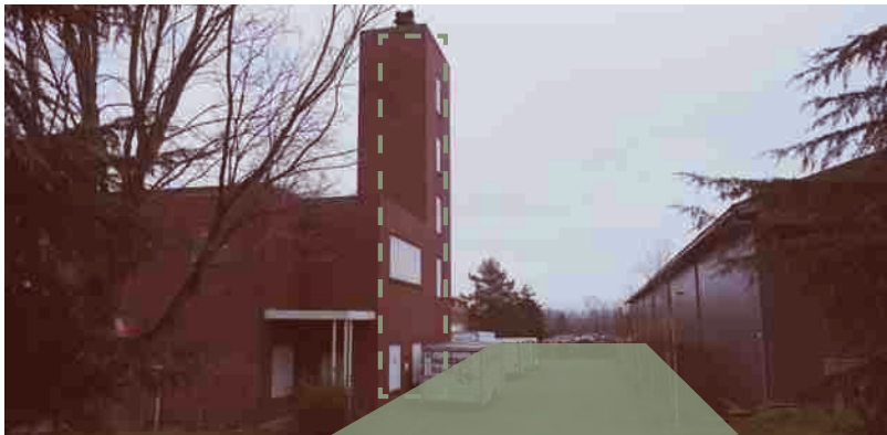
Figure 50. Back Alley between building 18 and the Tennis Center
