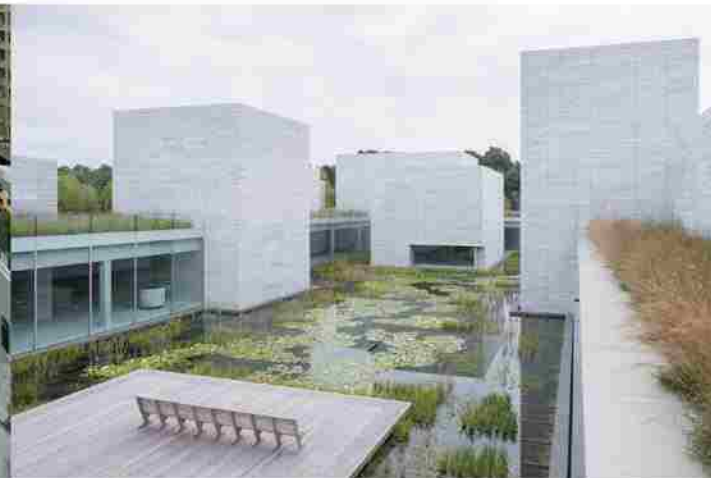
Figure 7. Glenstone Museum in Potomac, Maryland, USA | Thomas Phifer and Partners, PWP Landscape Architecture. Photograph by Iwan Baan
