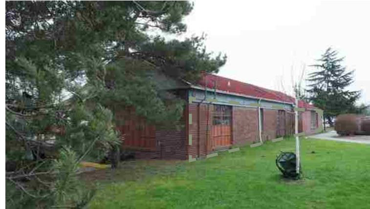
Figure 49. Significant feature - South facade of Building 41
