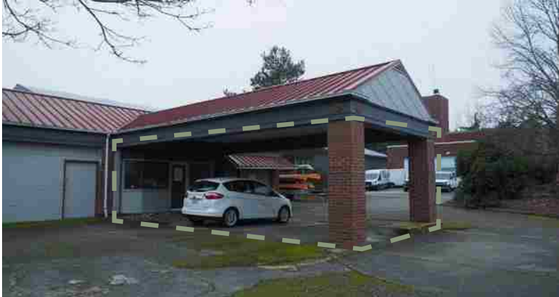
Figure 48. Significant feature - Porte cochere
