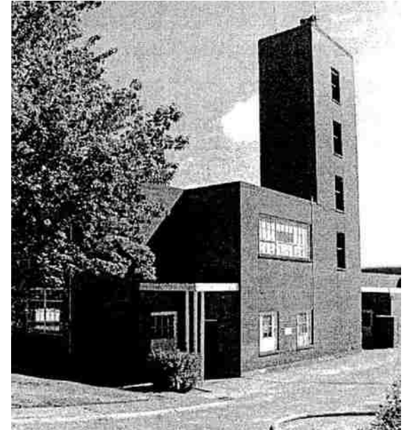
Figure 32. South side of the building. Source :Sand Point Magnuson Park Building 18 Firehouse Studio Project Feasibility Study Report By Arc Architects, page 10
