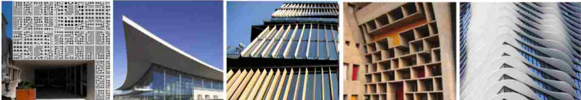
Figure 11: From left to right: Overhang-Gibraltar Airport by Blur Architecture and 3DReid, Louvers- Aqua was designed by Jeanne Gang, Fins-Asakusa Culture Tourist Information Center, Eggcrate-The Chandigarh High Court, Perforated Screen- Social Facilities in Roses by Exe arquitectura.
