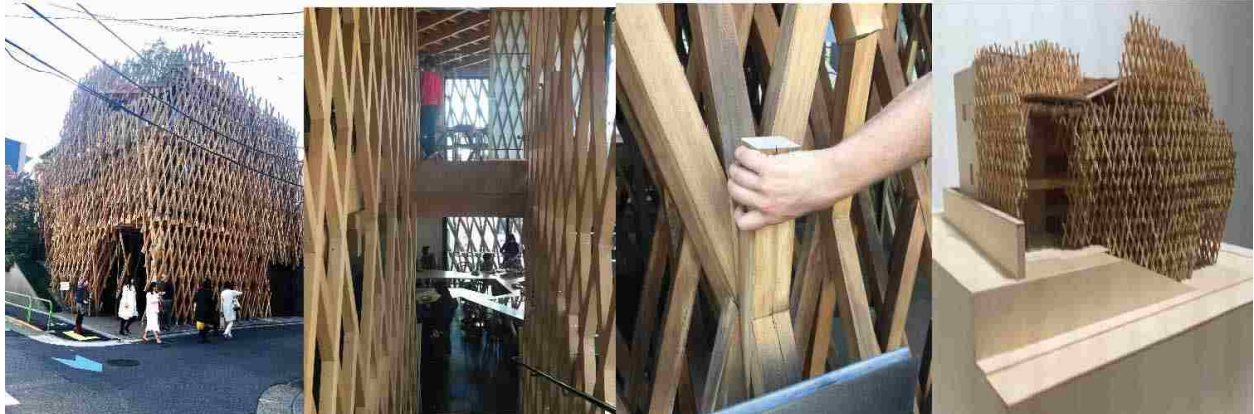
Figure 8. Sunny Hills in Site, Structure, Size of beam in Relation to Hand and Scale Model.
