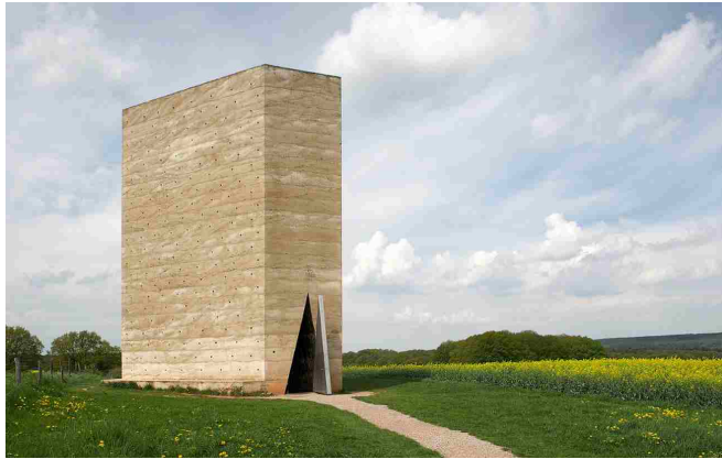
Figure 6. Bruder Klaus Field Chapel, Wanchendorf, Germany complete.
