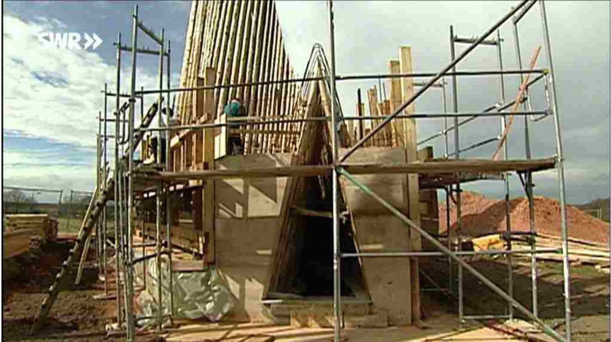
Figure 5. Bruder Klaus Field Chapel, Wanchendorf, Germany during construction.
