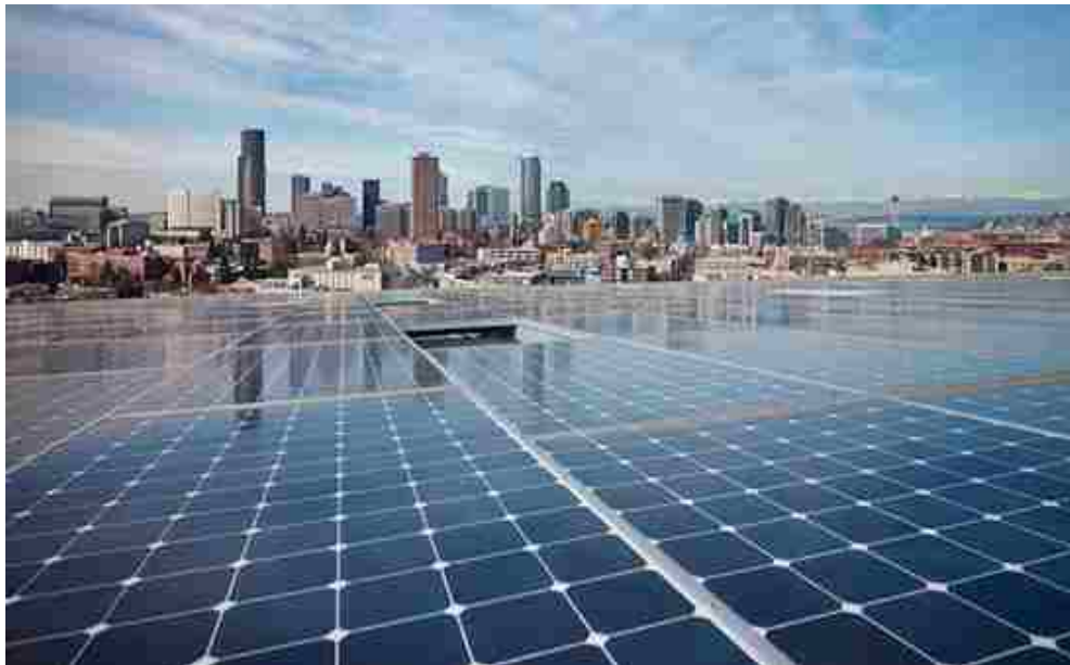
Fig.3. Bullitt Center Roof with 575 BIPV
