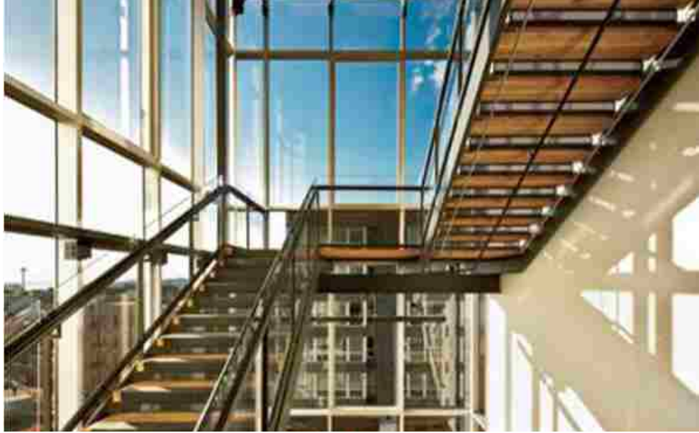
Fig.2: Bullitt Center staircase
