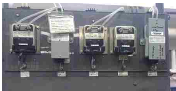
r. Airside Pressure Transducers Panel Mounting
