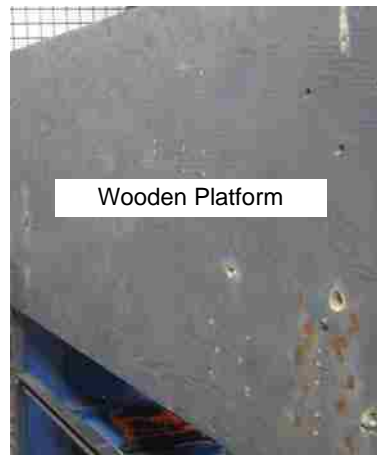
c. Liquid handling system panel construction-1
