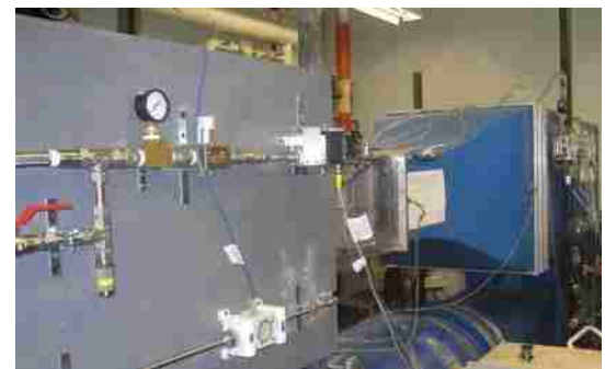
j. Liquid handling system panel construction-6
