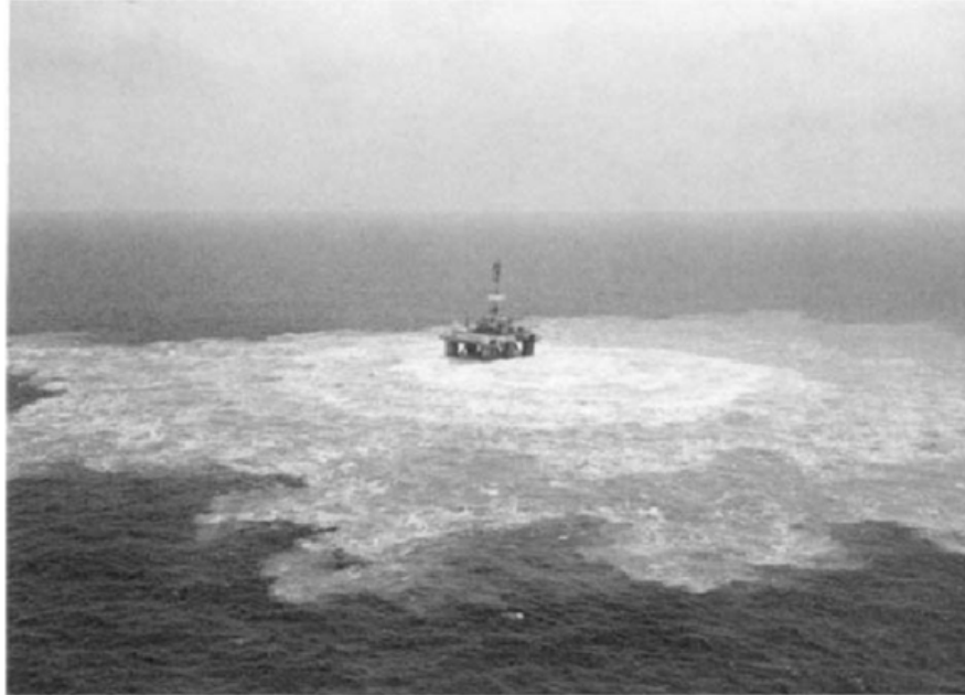
Fig. 2.2-Loss of subsurface well integrity in offshore well [14]
