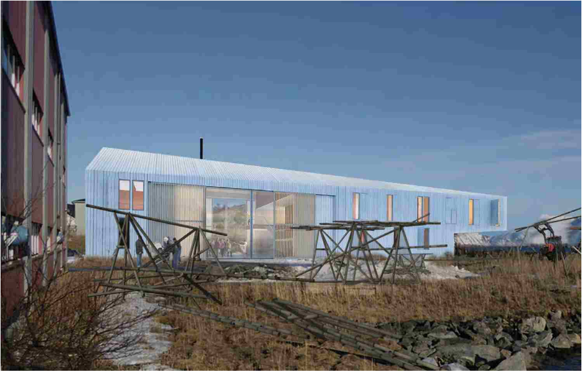
Figure 53: View north from southern extreme of site
