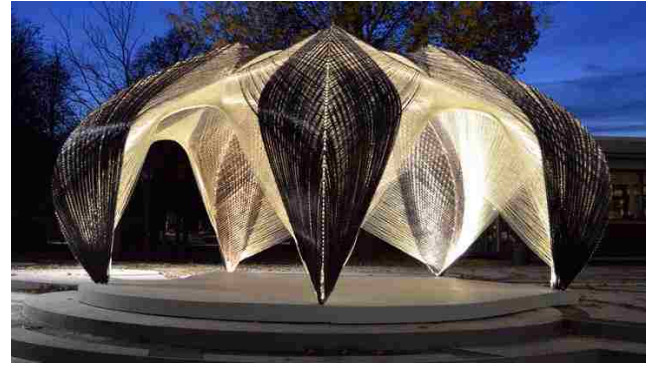
fig. 23 Monocoque carbon and glass fiber shell
