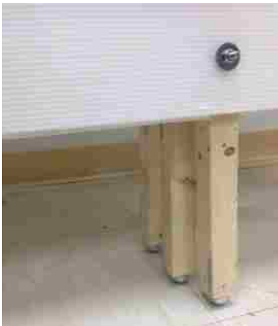
Figure 40 - Single ball caster for each panel's leg
