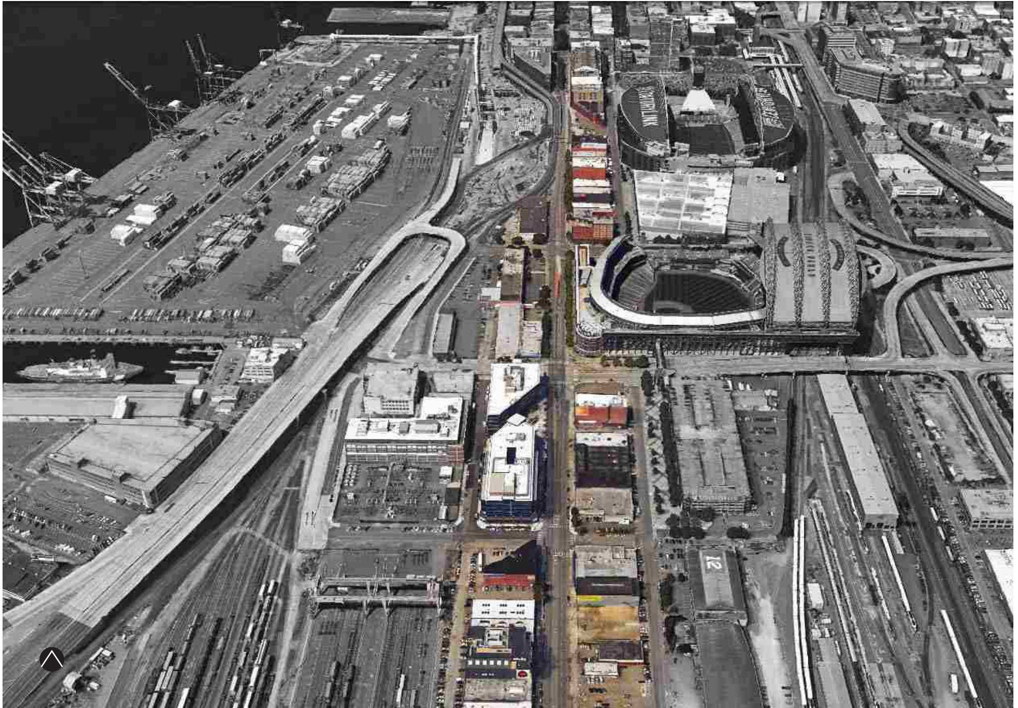
Figure 14. The streetscape of First Avenue South in SoDo; small-scale fabric mediating the commercial industries and entertainment industry
