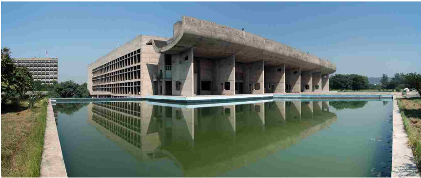
[fig. 30a] Palace of Assembly, Chandigarh, India
