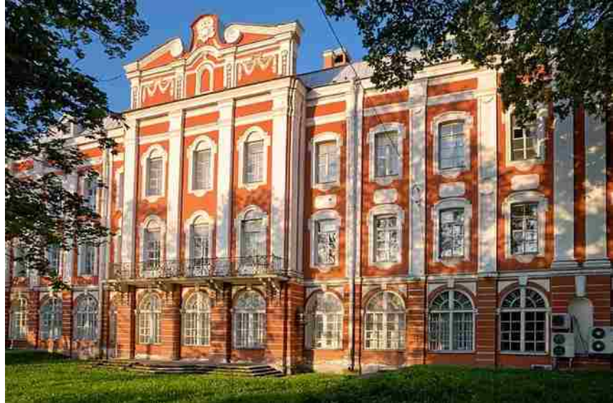
Figure 3.14 Building of the Twelve Colleges. Photograph showing the pedimented central bay of one of the twelve linked structures.
