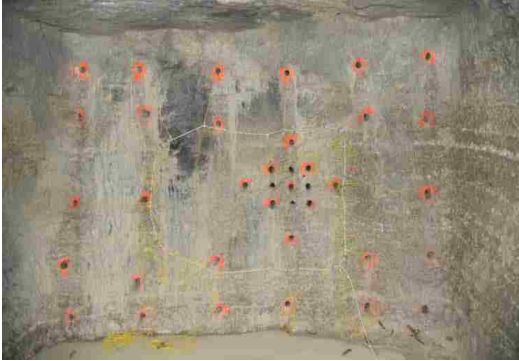
Figure 5.2. Representation of explosives and detonators loaded into holes
