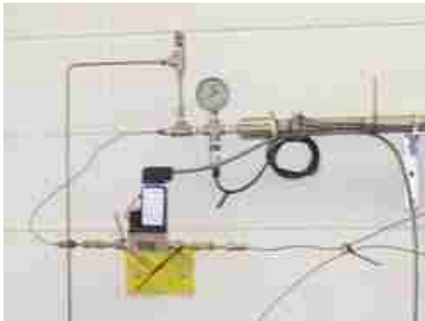
Fig. 3.4. Pipe inlet with upstream foam generator and gas flow meter
