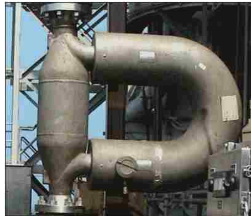
Fig. 2.5: Coriolis flow meter (With the permission of AT BALANCE™)
