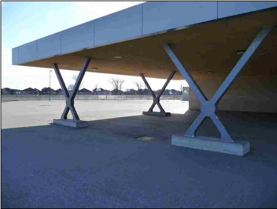
Figure 56. ES-09: Architectural design that attached a large roofed space to main school building.
