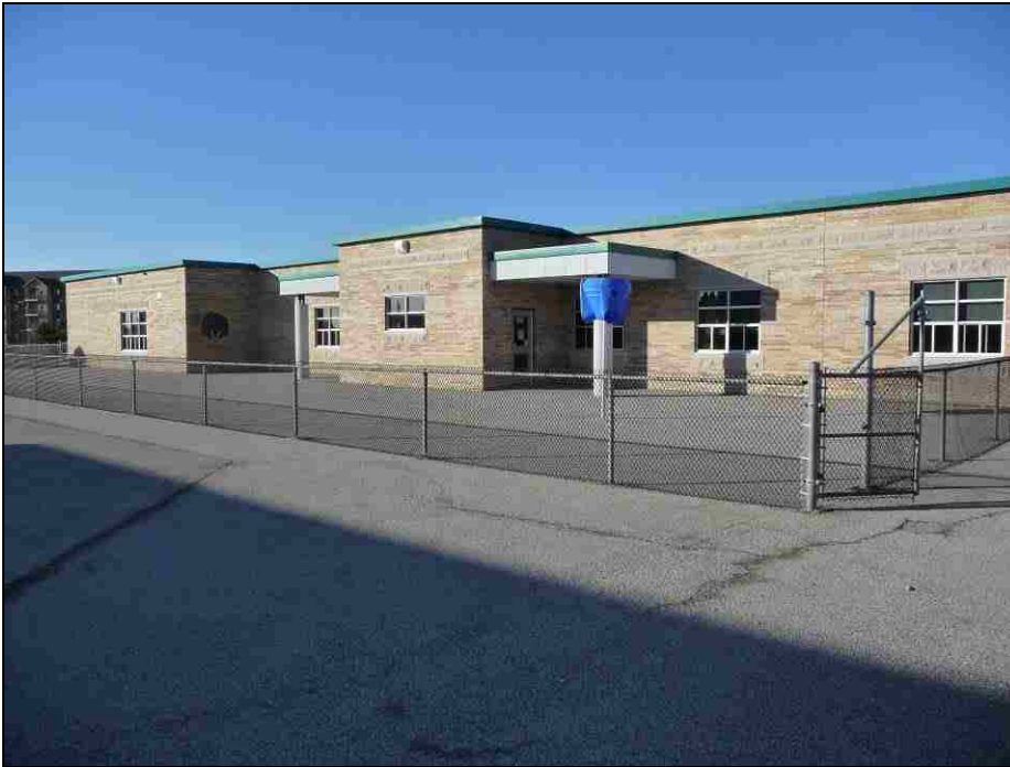
Figure 43. ES-02: Combination of school building walls and a chain link fence provide important security elements for young children.
