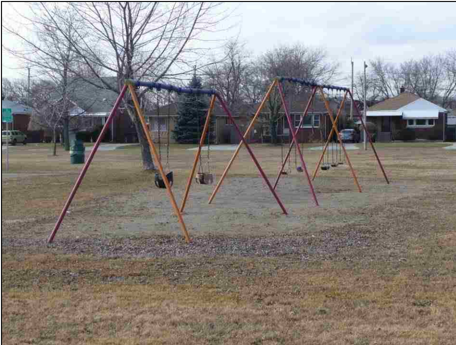
Figure 33. ES-04: Traditional swing set constructed of steel tubing.
