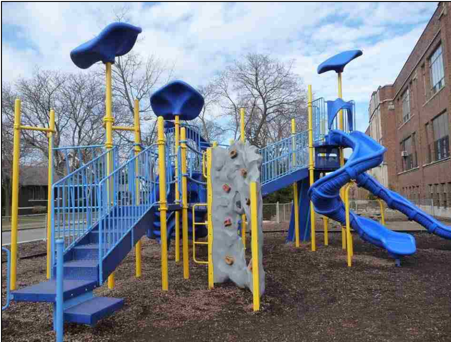
Figure 16. ES-05: Superstructure fabricated from metal/plastic and placed atop woodchip ground cover.
