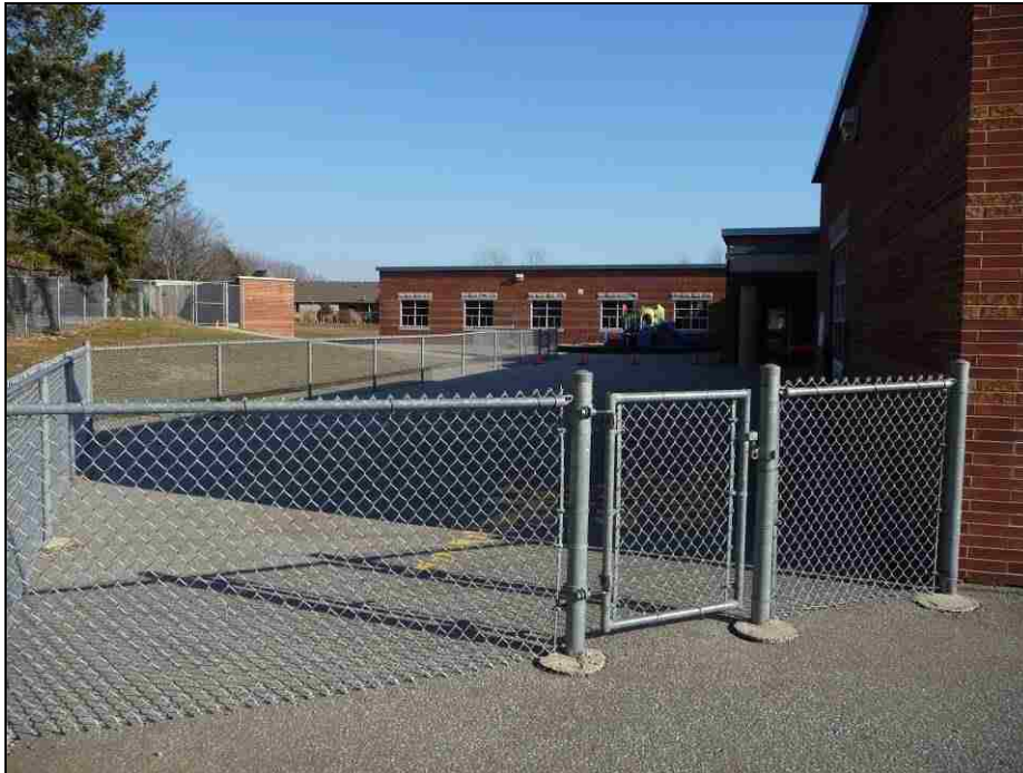
Figure 46. ES-08: The schoolyard and playground are partitioned using structural features of the school building and a chain link fence.
