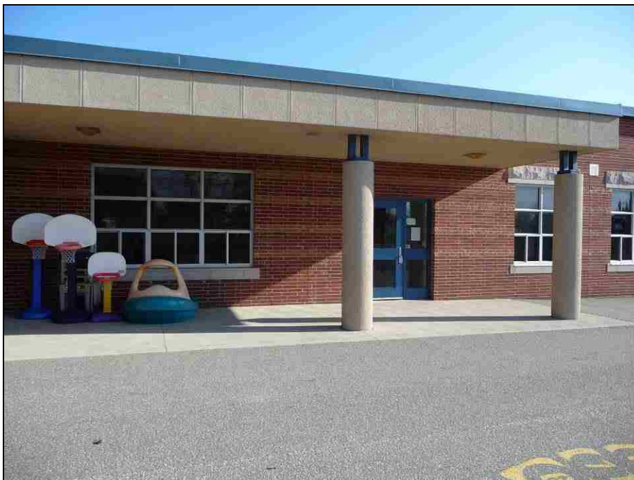
Figure 55. ES-08: Overhang along school building provides children with protection from the weather.
