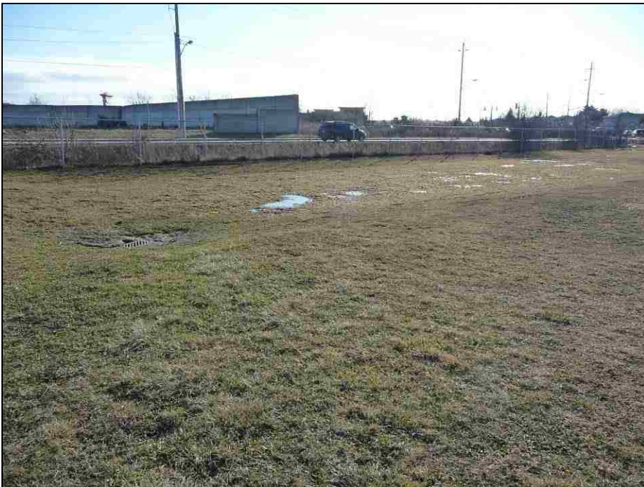
Figure 72. ES-10: Flooded area of schoolyard.
