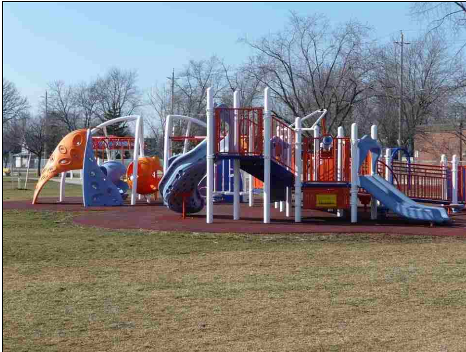
Figure 17. ES-07: Superstructure made using metal/plastic components and situated atop a synthetic rubber surface.
