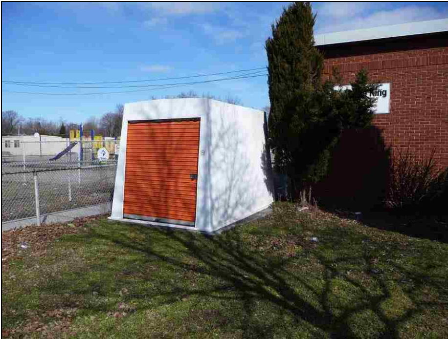
Figure 59. ES-06: Storage locker located adjacent to playground equipment.
