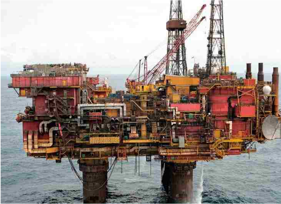
Figure 1.2: A typical offshore platform
