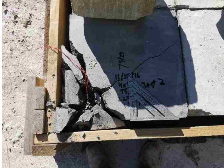
Figure 24 Surface Breakage Test 16
