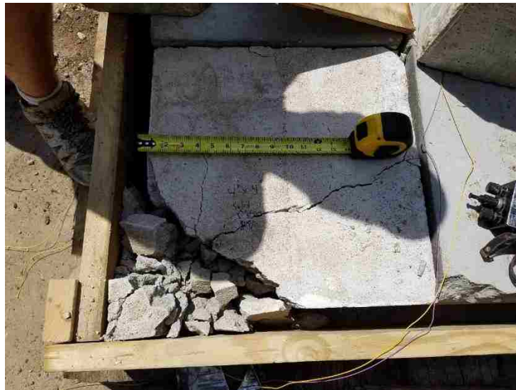
Figure 9 Surface Breakage Test 5
