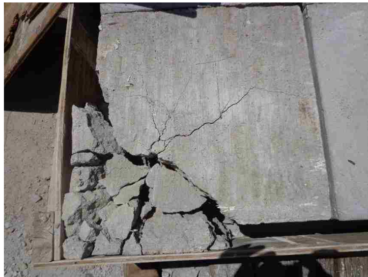
Figure 5 Surface Breakage Test 3
