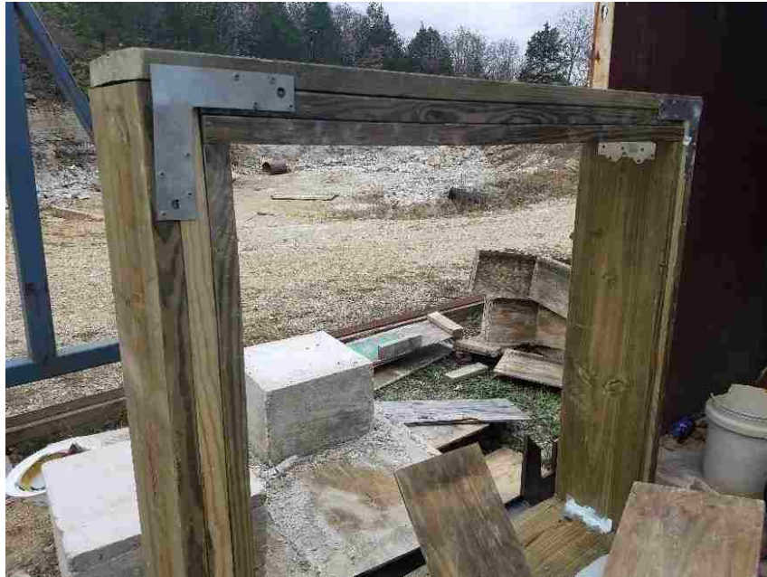
Figure 4.5. Reinforced Crib Construction
