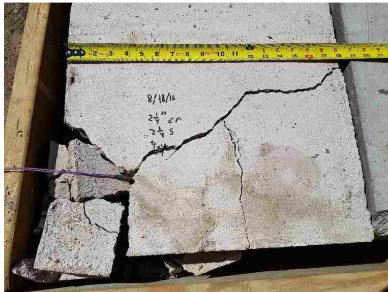
Figure 13 Surface Breakage Test 7
