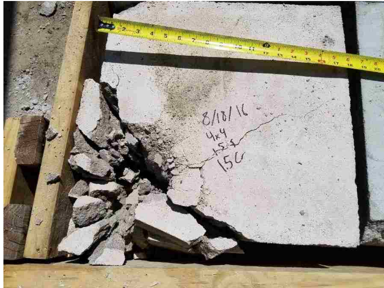
Figure 18 Surface Breakage Test 10
