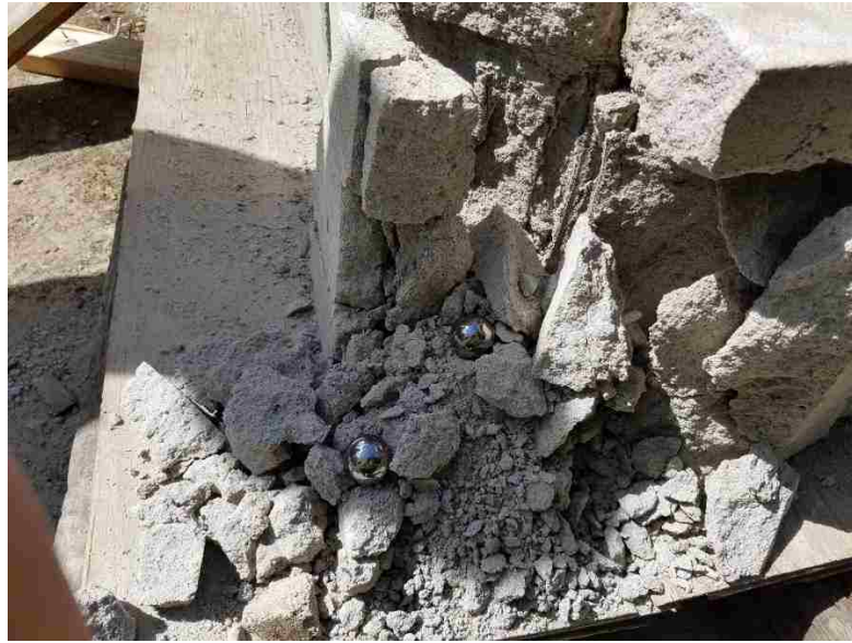
Figure 14 Substrate Breakage Test 7
