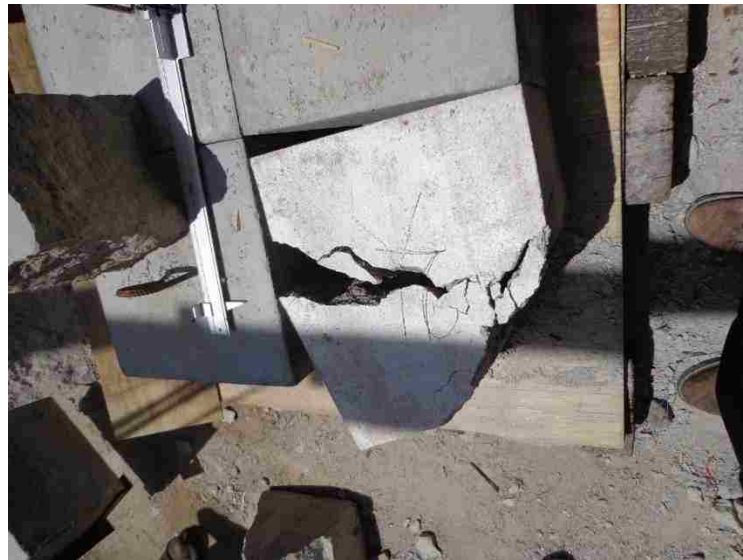
Figure 7 Surface Breakage Test 4
