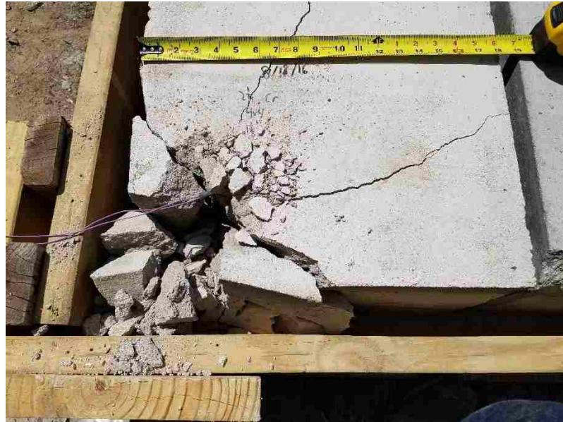
Figure 16 Surface Breakage Test 8
