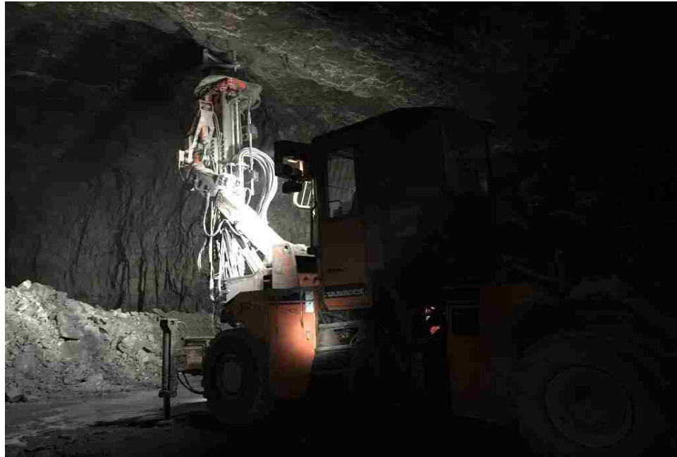
Figure 3.4 Roof drilling operation in the mine Z
