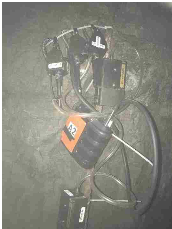
Figure 3.6 DPM monitors installed in the mine Z
