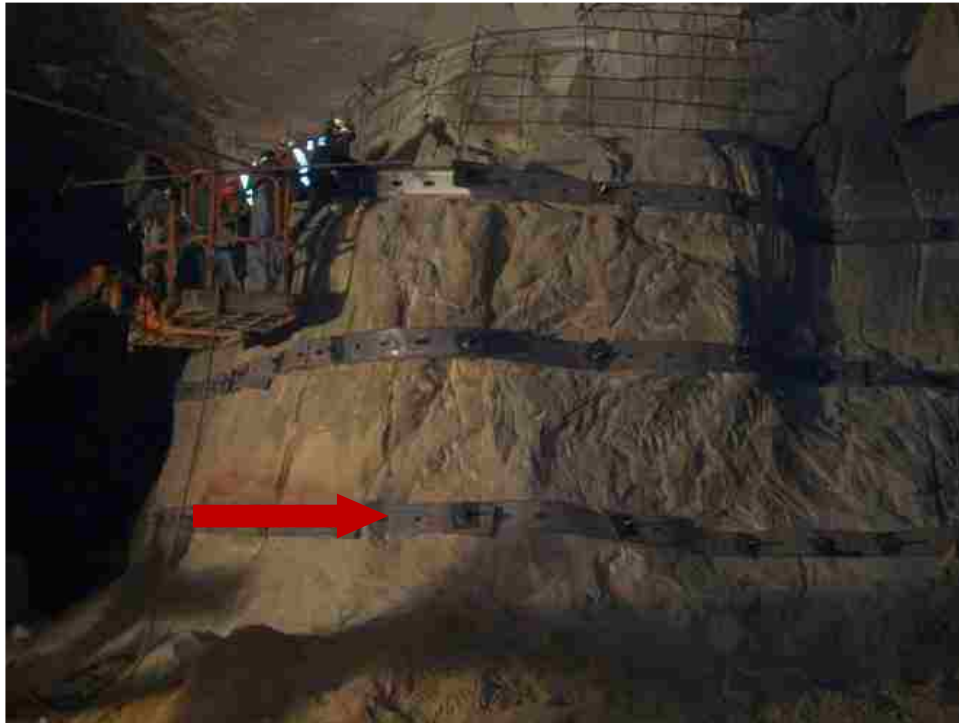
Figure 1.4. Reinforcing a sandstone pillar with rockbolts and steel strips.
