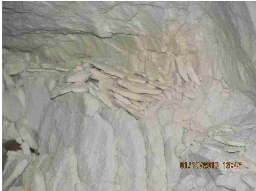
Figure 4.17. A close look of at initial pinch-out failure formation
