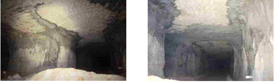
Figure 4.45. Stopping initial failures by applying a thin layer of shotcrete.
