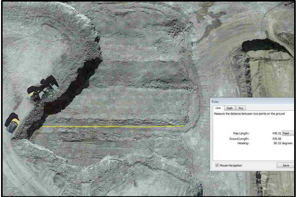
Figure 3.4: Cloud Peak Energy Antelope Mine Bench Blast
