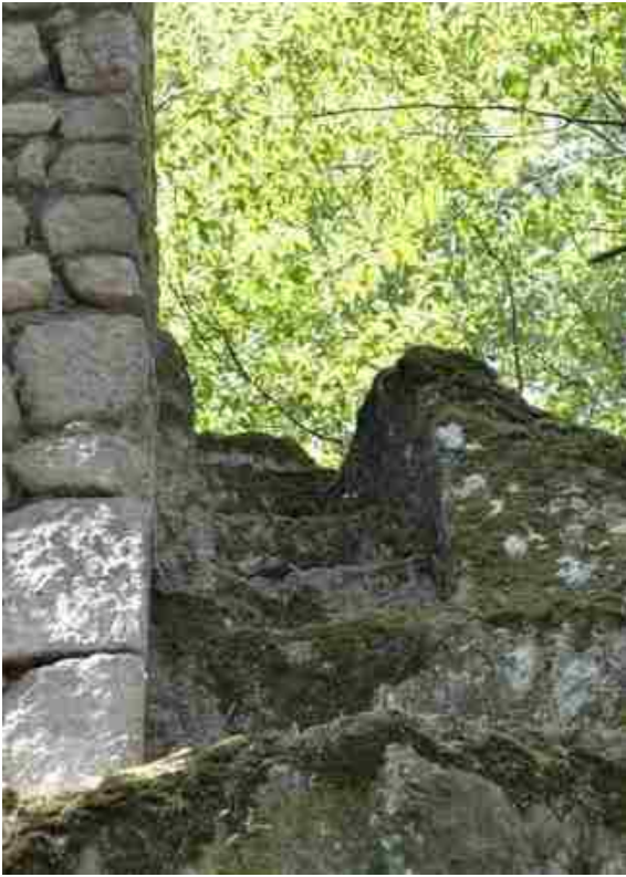
FIGURE 82 Brick tower, detail Sacro Bosco
