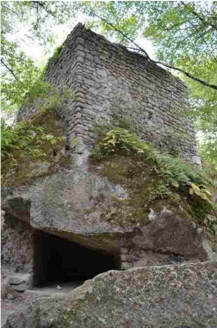
FIGURE 30 Brick tower Sacro Bosco
