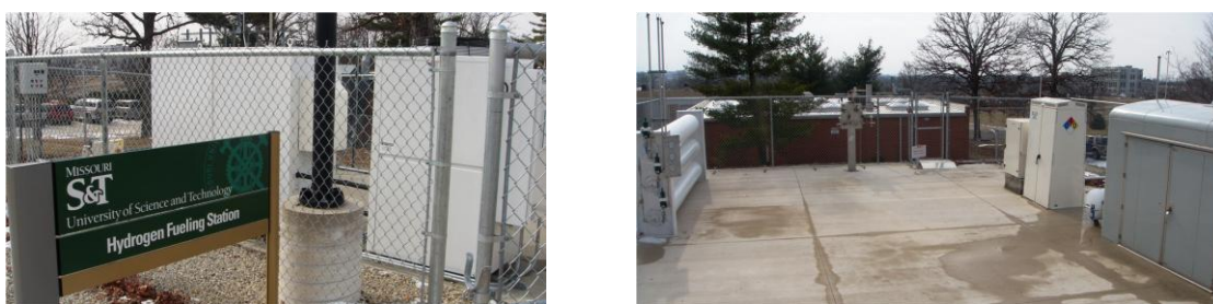
Figure 5 – Hydrogen fueling station
