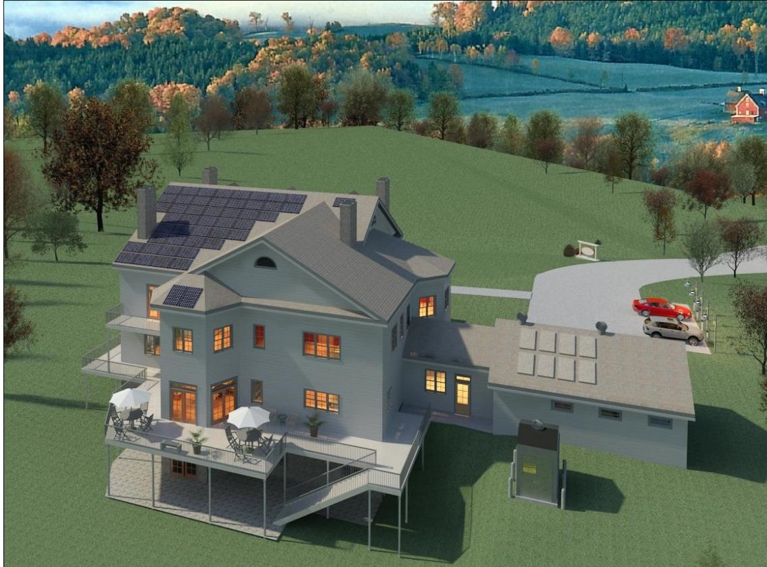
Figure 5. Bed & Breakfast in Wallingford, CT (solar panels, garage, and hydrogen storage)
