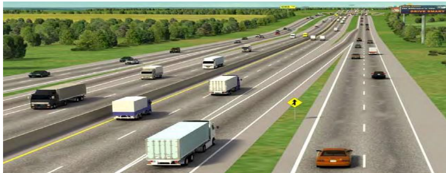
a) Proposed truck-only lane slip ramp configuration
