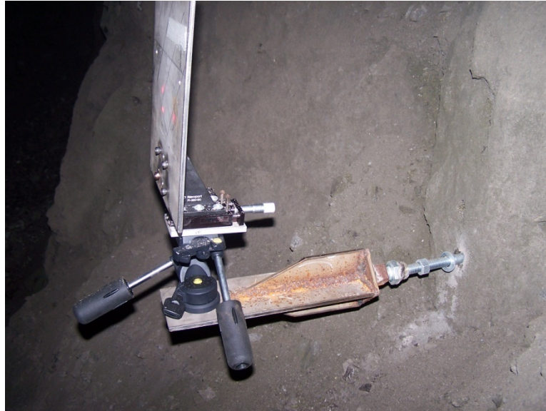
Figure 3.3: The target section of the HRTMM mounted on a rock anchor. The heavy-duty tripod head, aluminum plate, micrometer, right-angle bracket and stainless steel plate are visible from the bottom up.
