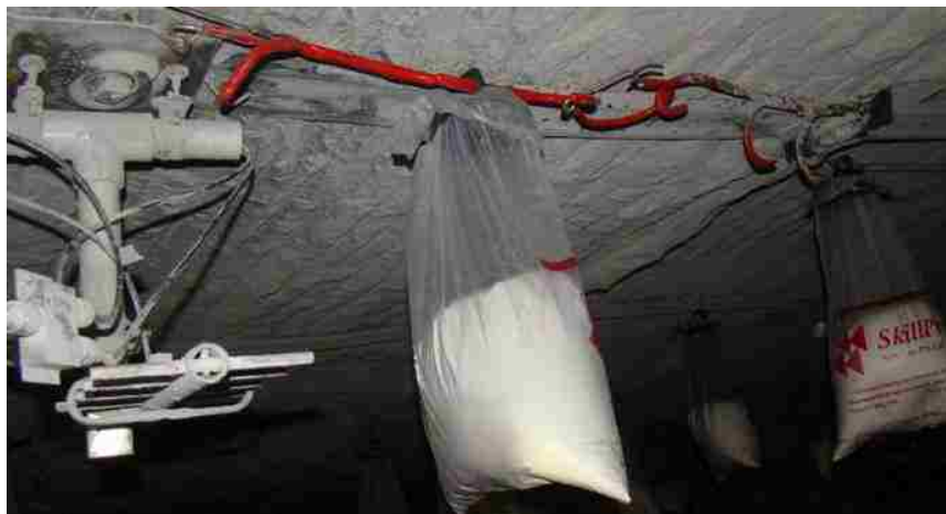
Figure 4.5: Rubber Coated Cable Hanger Support Method
