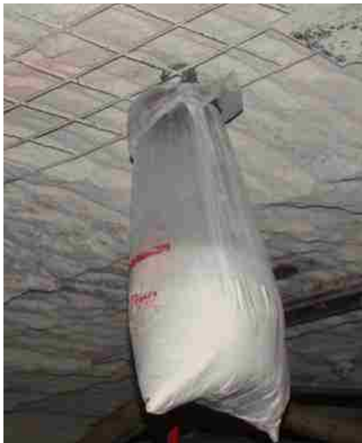
Figure 4.9: Barrier Bag Hung from Roof Mesh
