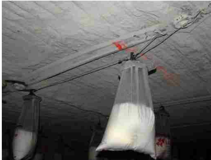
Figure 4.4: Cable and Hook Support Method
