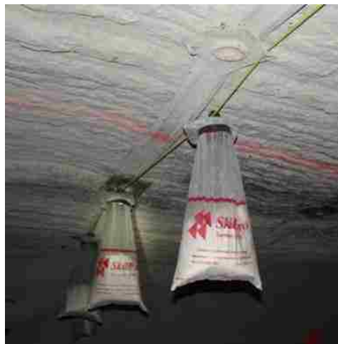
Figure 4.3: Bolt Plate/Cable Support Method
