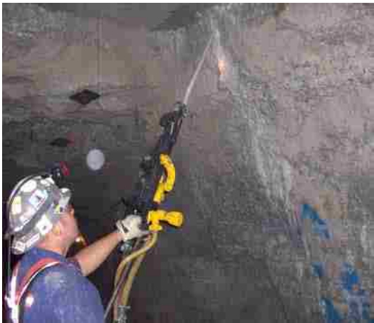
c. Drilling a Hole.
