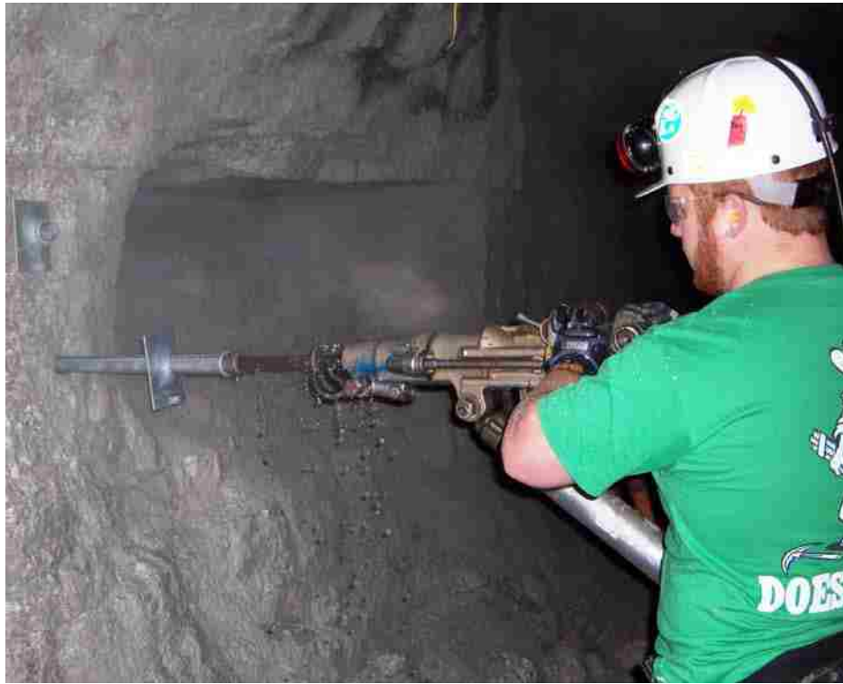
Figure 4.20. A Participant Installing a Split Set Rockbolt During the Underground Rockbolting Contest.
