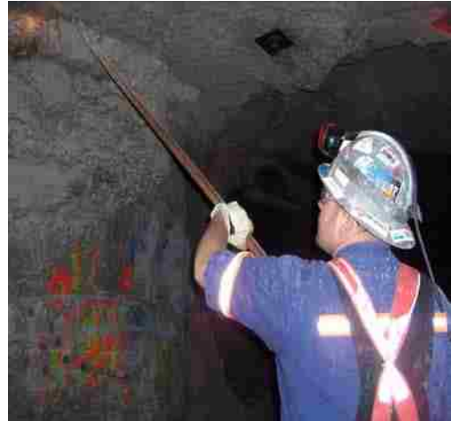
b. Scaling Loose Rock.
