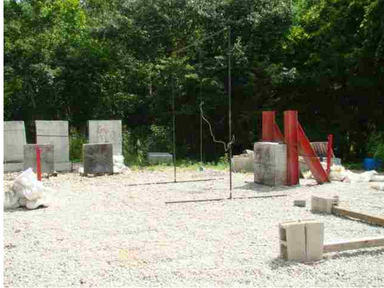
Figure 6.1 Barrier chained to supporting I-beams
