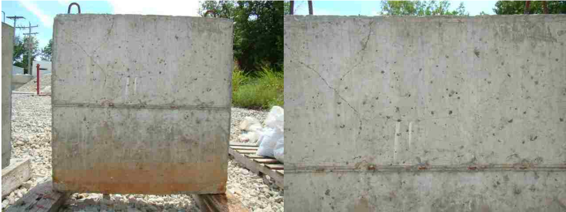
Solid concrete barrier
