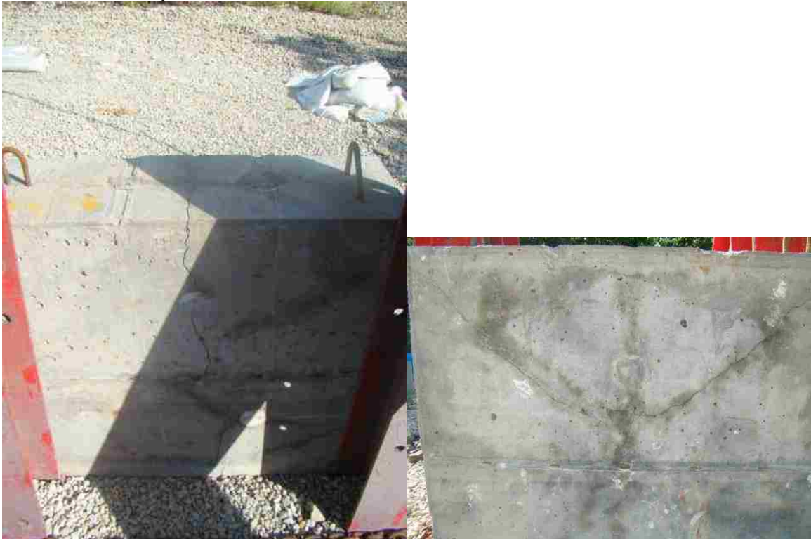
Barrier with cavity no LCFs
