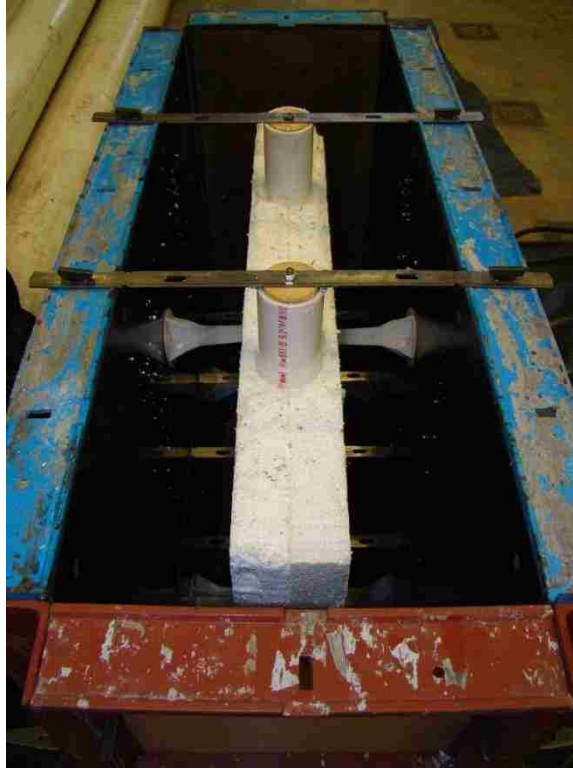
Figure 3.7 Frame and foam secured and ready for pour
