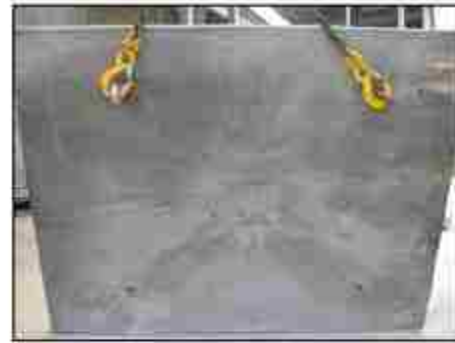
Panel 4 (conventional reinforced concrete) front surface after explosion - Slight cracks
