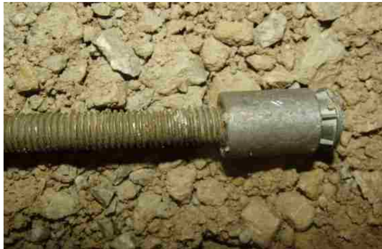
Figure 3.9. An Example \frac{1}{2} - 13 Ready Rod and Korker
