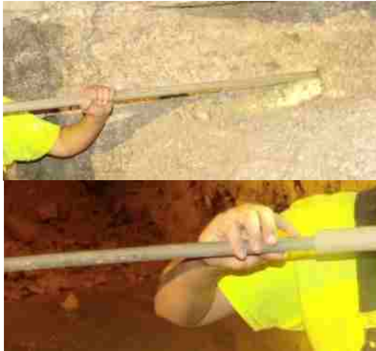
Figure 3.15. Measuring Pole in Use
