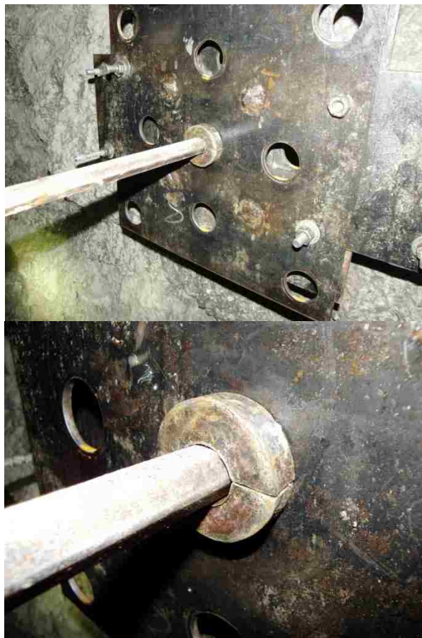
Figure 3.11. Inserting the Split Collet and Leveling the Steel
