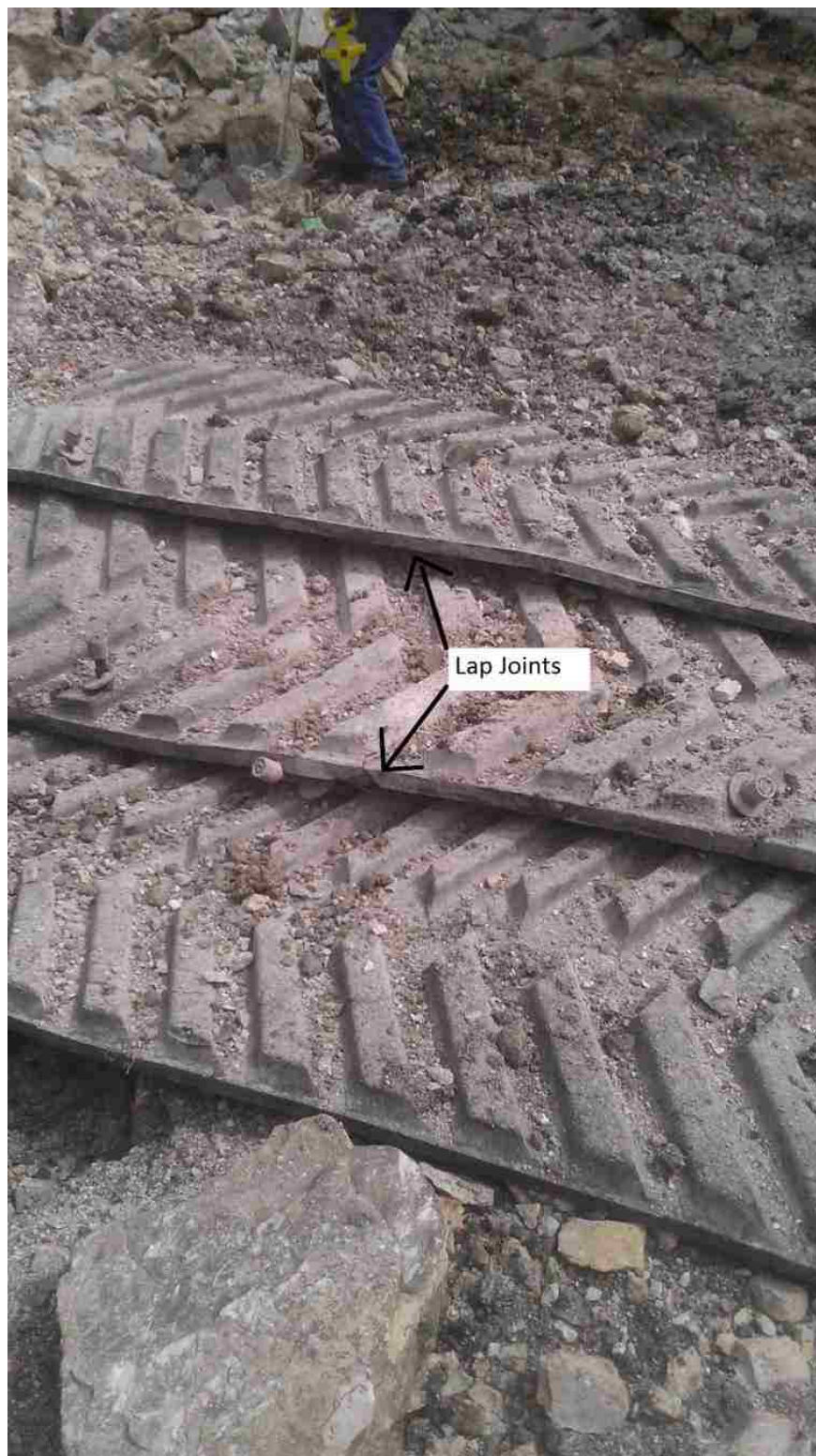
Figure 4.5 Tractor Tread Lap Joints
