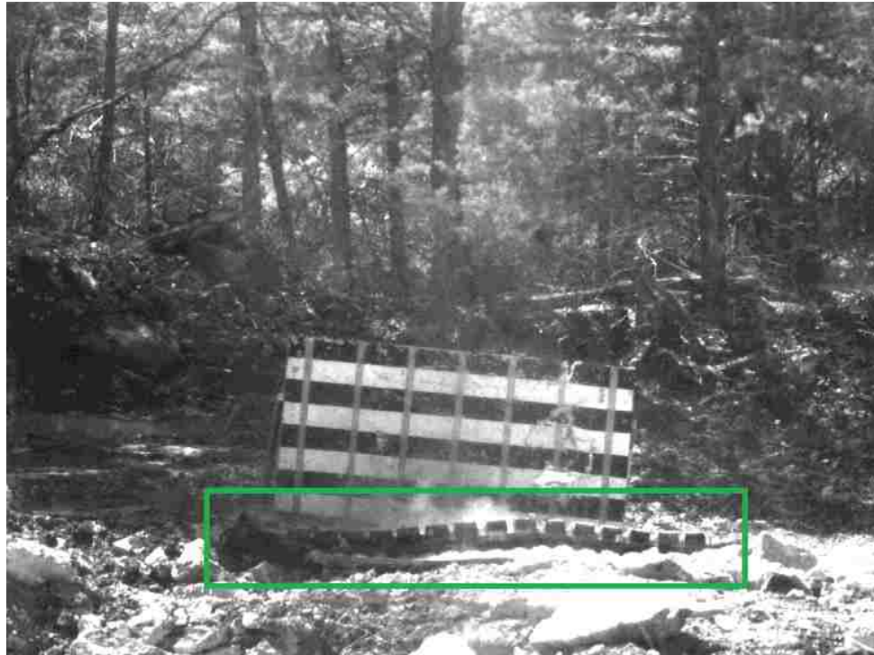
Figure 6.1 Blasting Mat Centered Over Borehole
