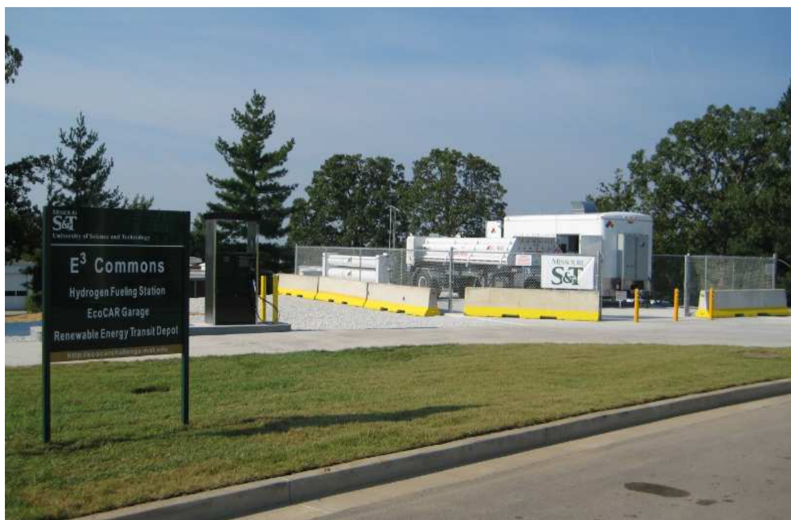
Figure 2.1. Missouri S&T Hydrogen Fueling Station at E 3 Commons
