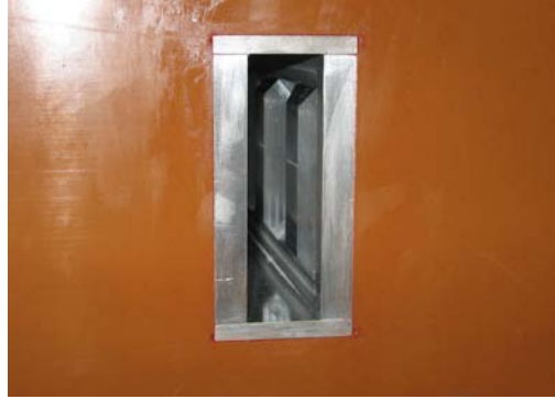
Figure 3.33: Silicone added to fill any voids
