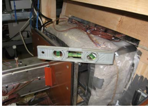
Figure 3.35: Leveling phenolic flange to match aluminum flange
