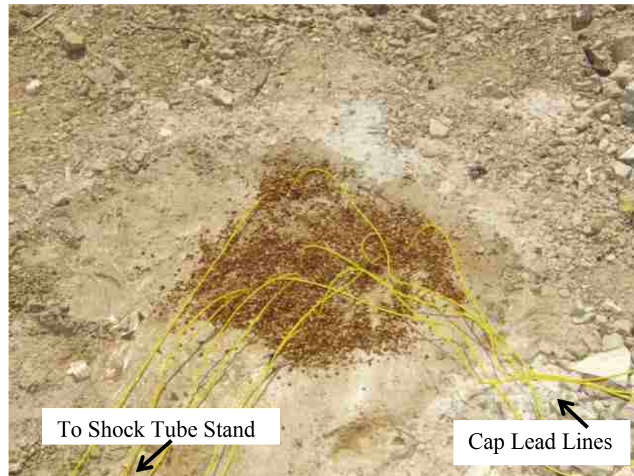
Figure 3-7: Top View of Loaded Holes
