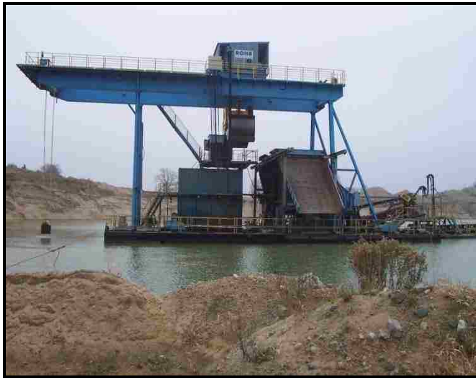
Figure 1.1 Clamshell dredge on site
