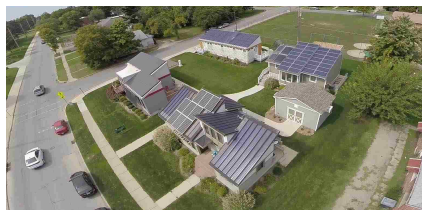
Figure 1. Solar Village at Missouri S&T.
