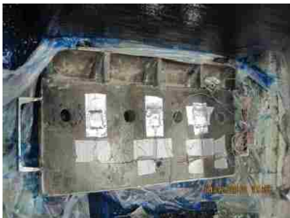
(a) Temporary Placement of Anchorage Over “Wet” Saturant
