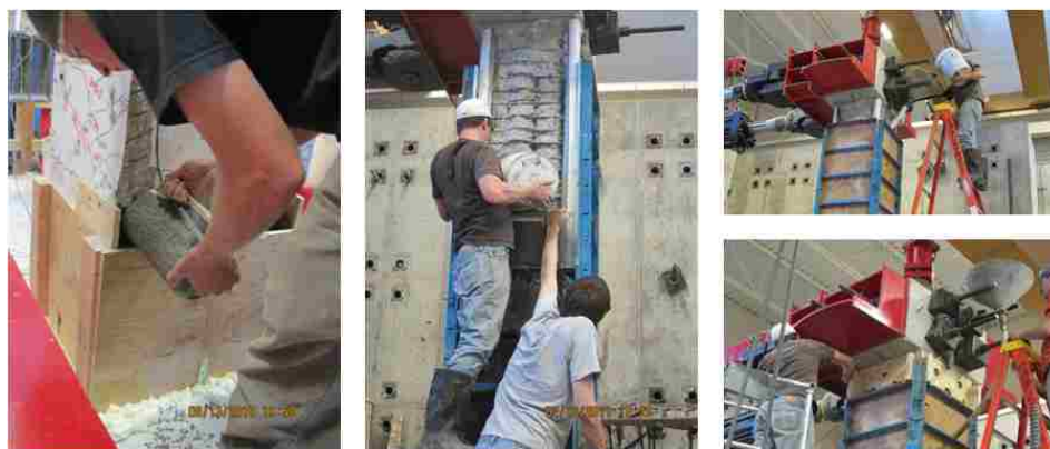
Figure A.4. Placement of Repair Mortar
