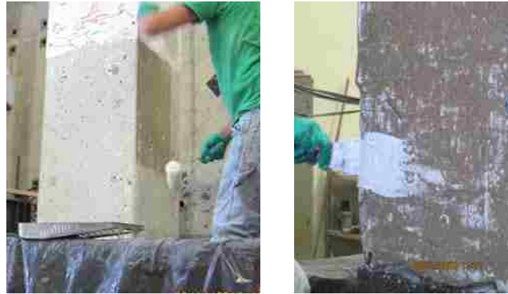
(a) Application of MBrace® Primer (b) Application of MBrace® Putty
