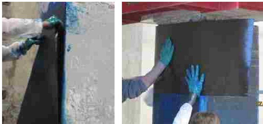
(a) Application of Longitudinal CFRP (b) Application of Transverse CFRP
