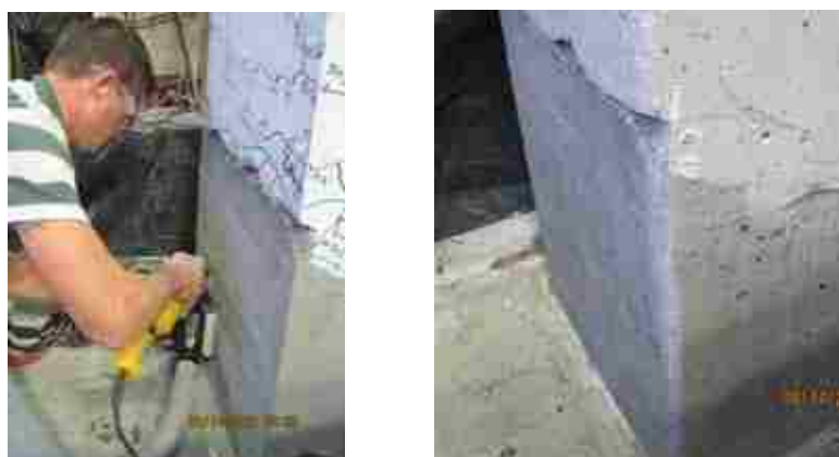
(a) Smoothing Concrete Surface
