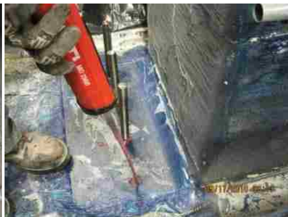
(b) Injecting Epoxy Into Anchor Rod Holes
