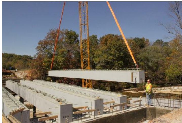
Fig. 2. B0439, HCB Erection Process
