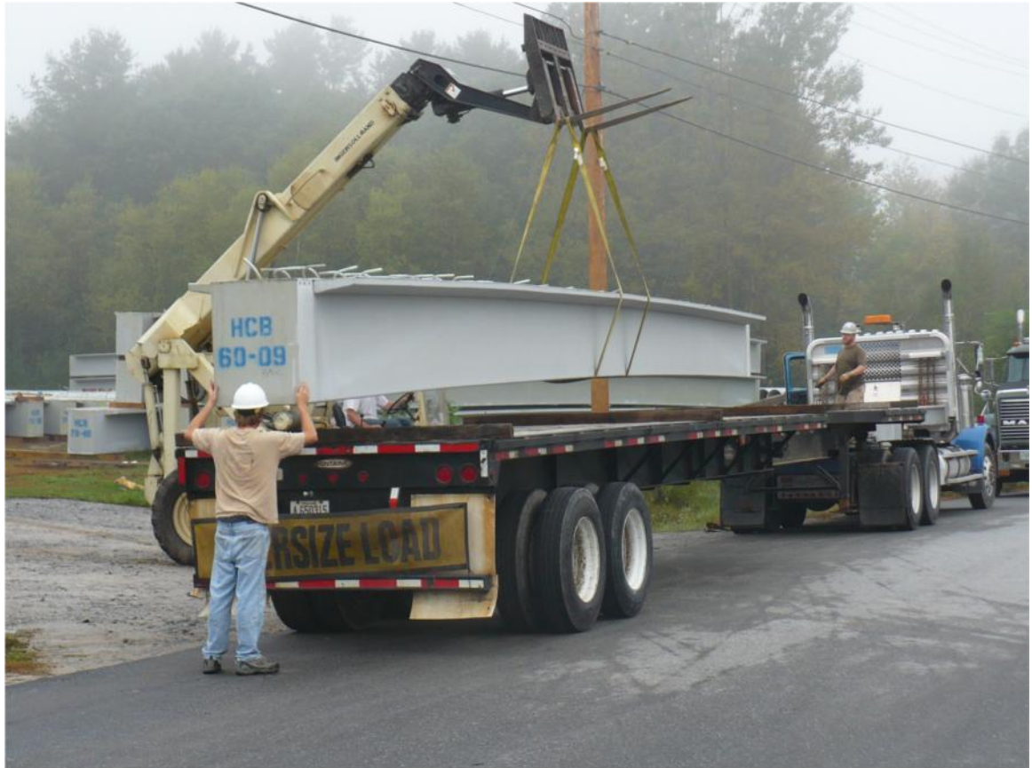
Figure 1.7. Loading of HCBs via small crane
