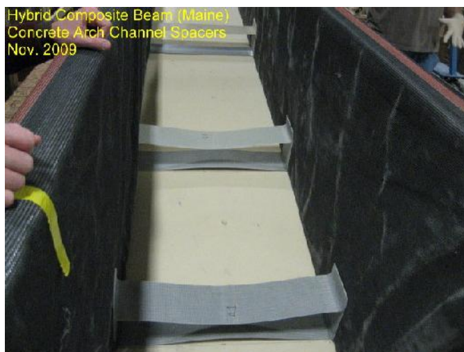
Fig. A-5. Spacer's installation
