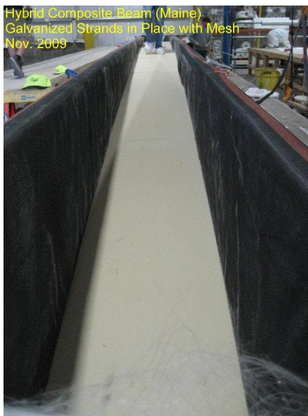
Fig. A-4. Placement of the lower foam blocks inside the box
