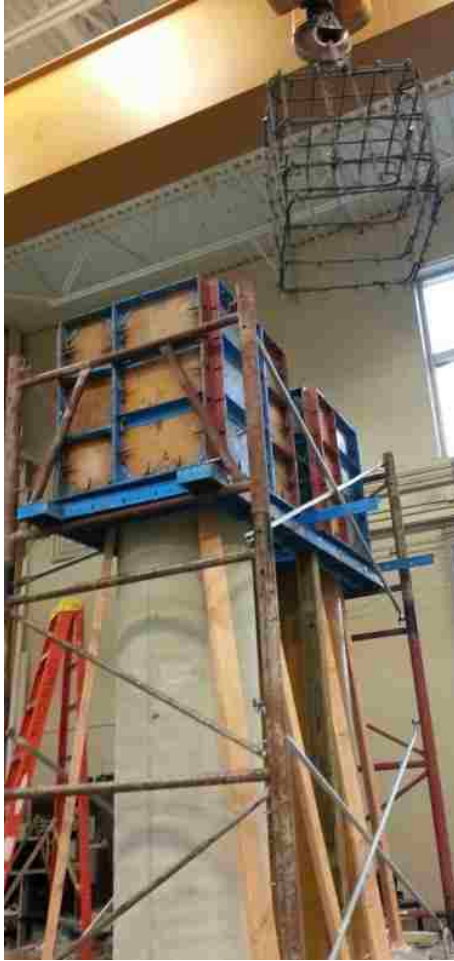
Install reinforcement cage
