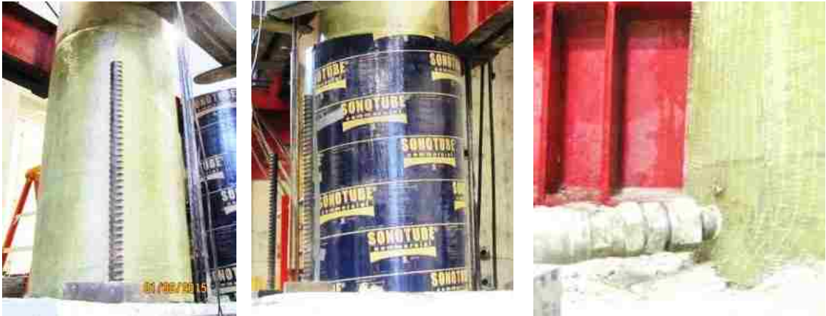
Fig. 2. Rapid repair of the C1 column: (a) wrapped GFRP, (b) heat chamber, and (c) grout injection
