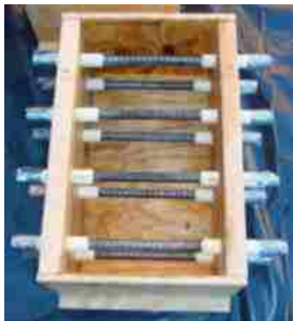
Figure 3.3 Mold to cast concrete block.
