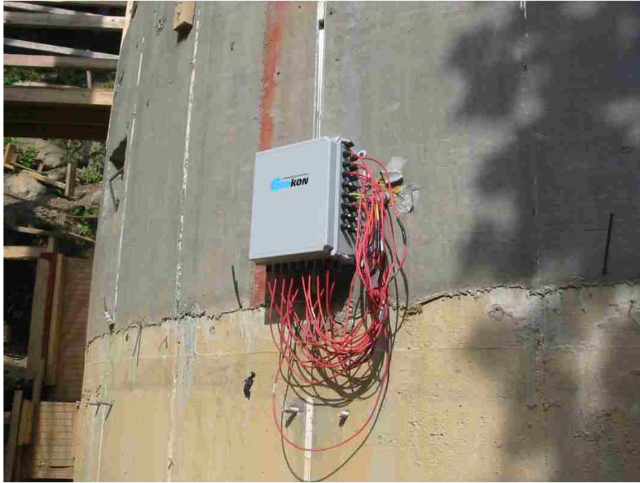
Figure 6.11. Photograph of Installed Terminal Box (Step 7)
