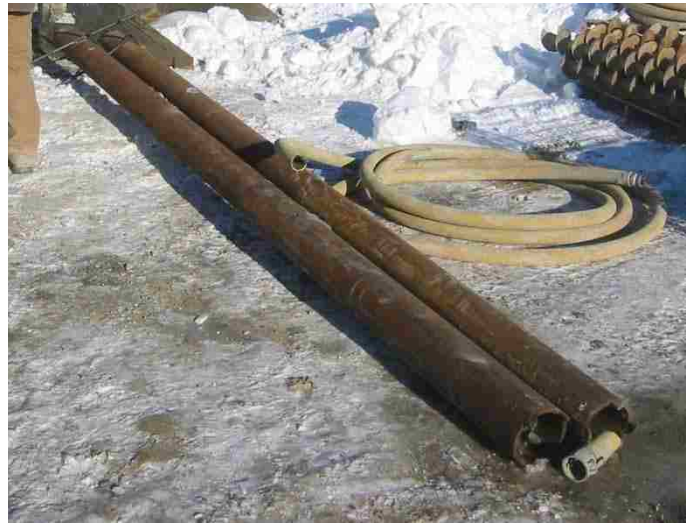
Figure 5.17. Micropile Casing (Steps 2 and 3)
