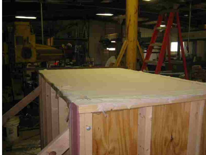
Figure 4.12. Photograph of Final Surface of Filled Sand Test Pit
