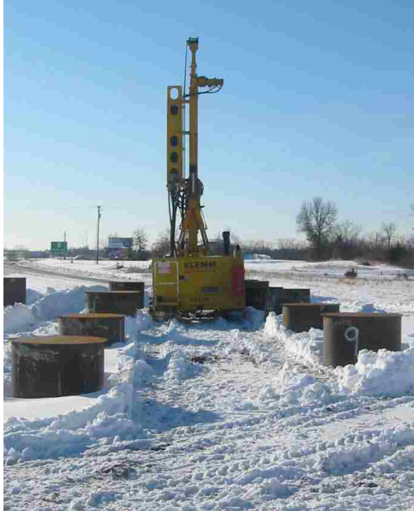
Figure 5.16. Micropile Drilling (Step 1)
