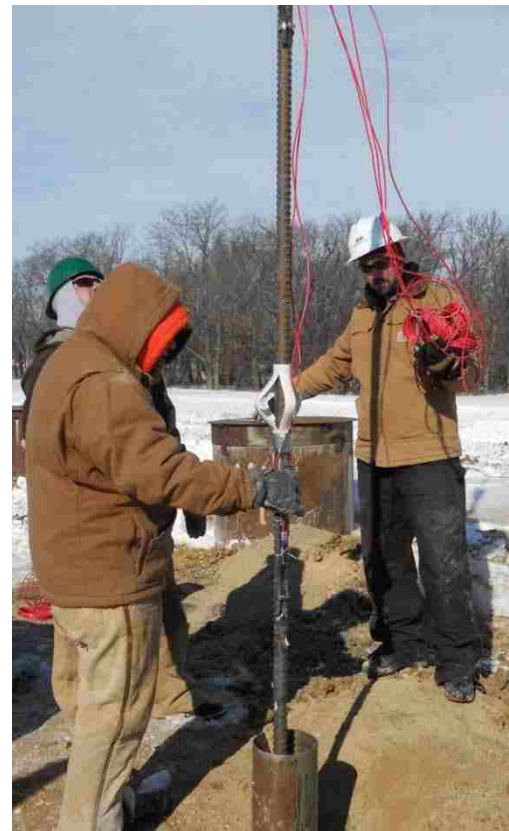
Figure 5.21. Placement of Central Reinforcing Bar (Step 7)
