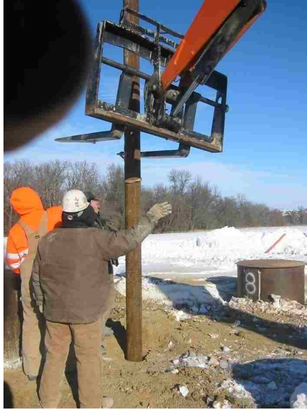
Figure 5.18. Installation of Micropile Casing (Step 4)
