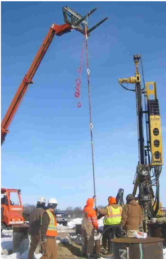
Figure 5.21. Placement of Central Reinforcing Bar (Step 7)
