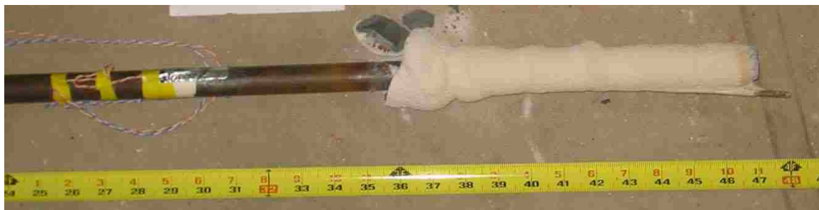
Figure 4.25. Photograph of Exhumed Pile 1B Bond Zone
