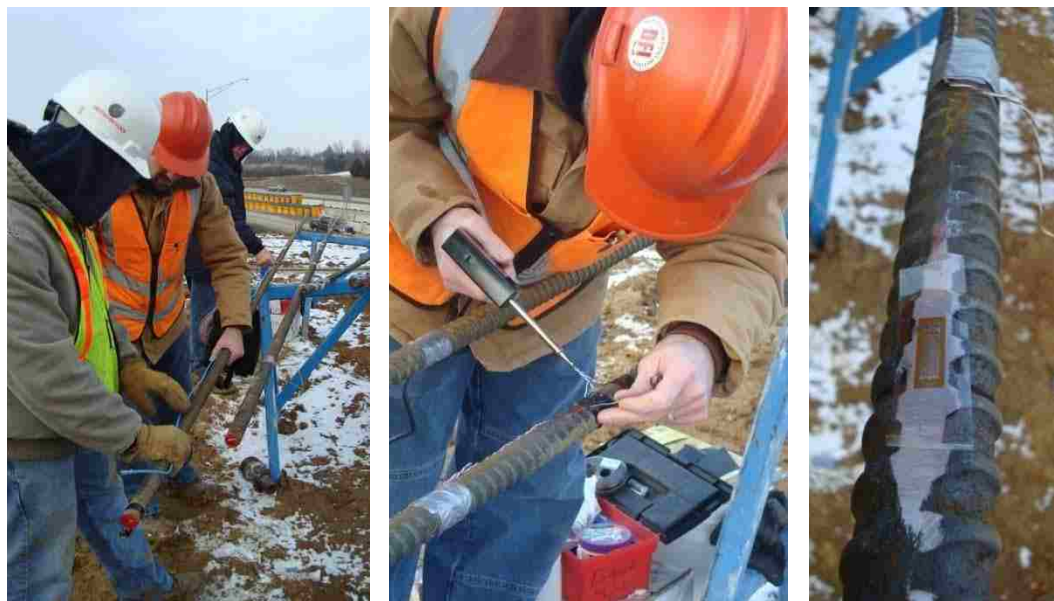
Figure 3.10. Photographs of Strain Gage Installation
