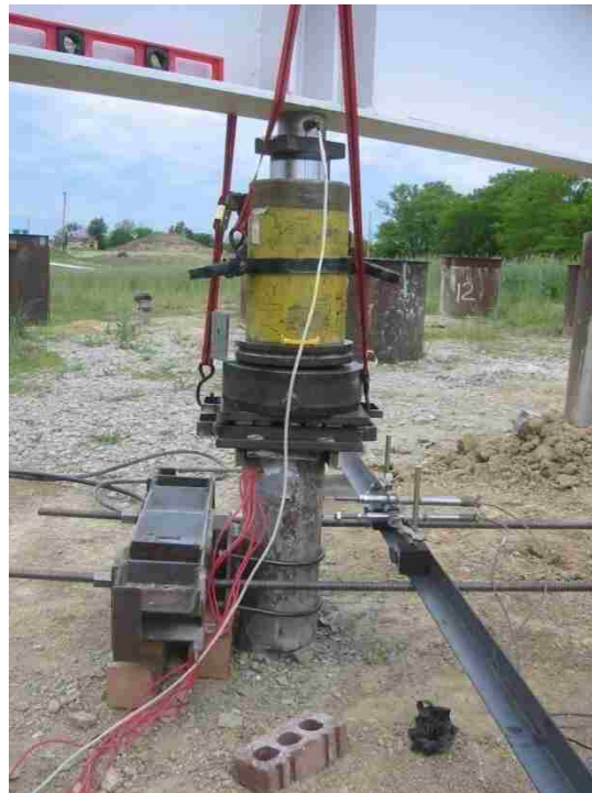
Figure 5.26. Combined Load Test
