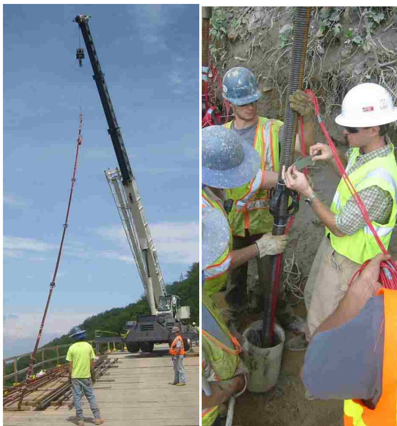
Figure 6.8. Photographs of Central bar Installation (Step 4)
