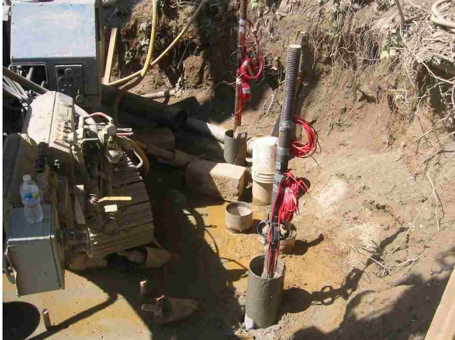
Figure 6.9. Photograph of Grouted Micropiles (Step 5)
