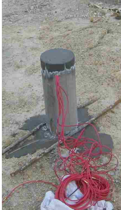
Figure 5.22. Final Grouting (Step 8)
