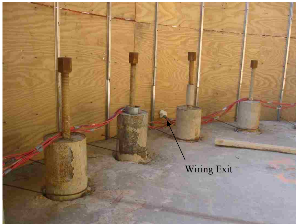
Figure 6.10. Photograph of VWSG Wire Routing through Pile Cap (Step 6)
