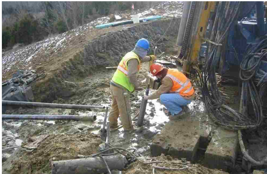
Figure 3.9. Photographs of Completed Micropile 58-G
