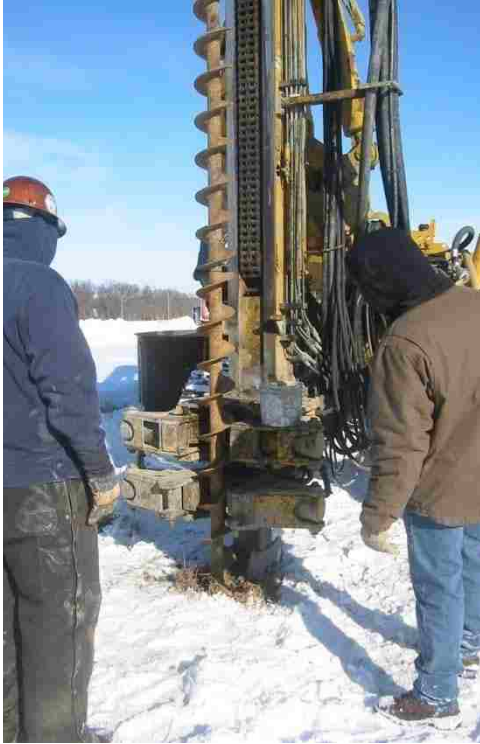
Figure 5.16. Micropile Drilling (Step 1)
