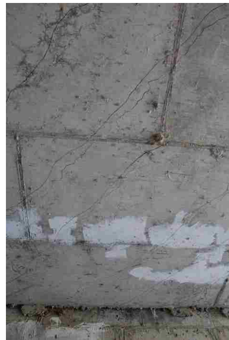
Figure 5.17. The cracks of span 4
