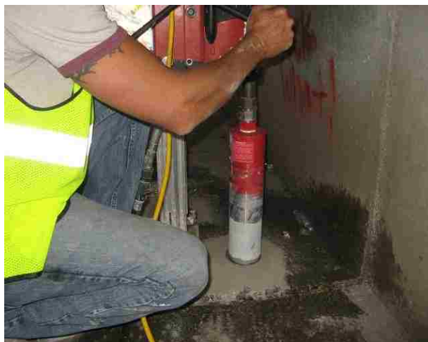
Figure 5.32. Concrete core extraction from Walker Bridge
