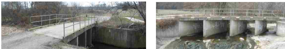
Figure 5.6. View of the existing Southview Bridge [120]
