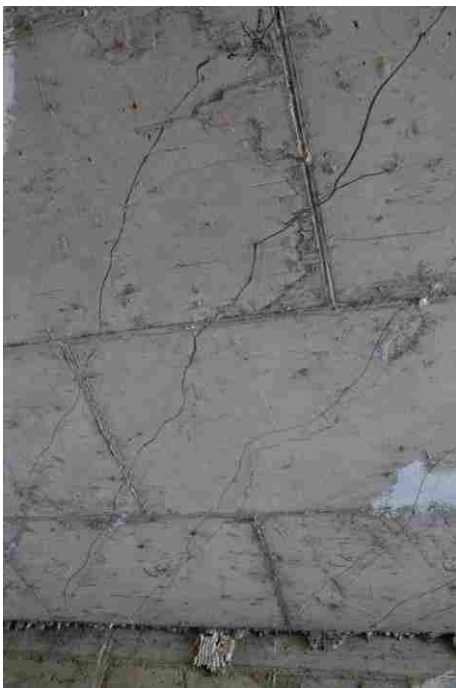
Figure 5.17. The cracks of span 4
