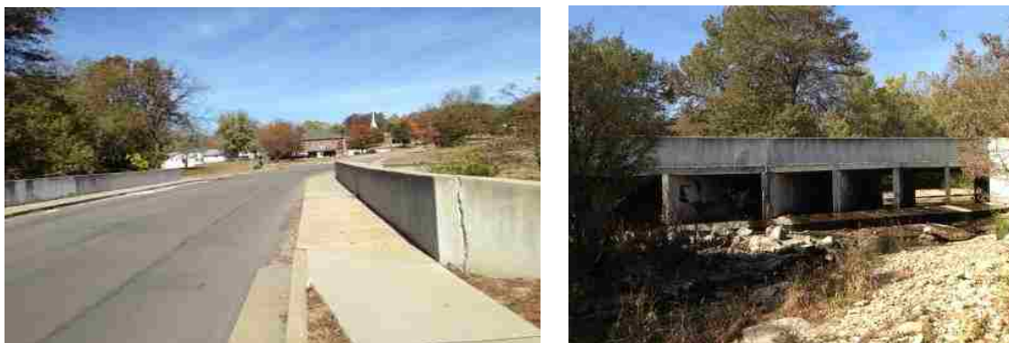
Figure 5.7. View of the new structure
