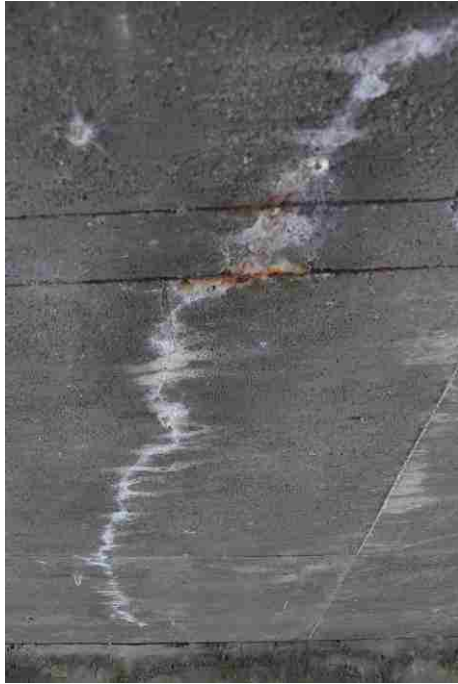
Figure 5.18. The cracks of span 5
