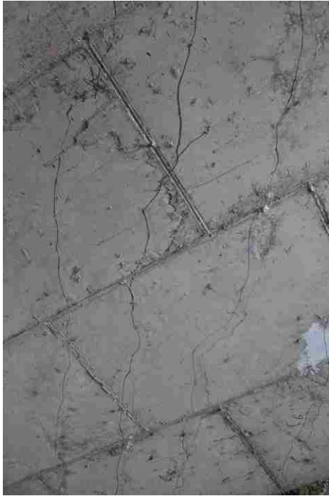
Figure 5.16. The cracks of span 3
