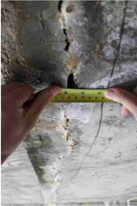
Figure 5.14. The cracks of span 1
