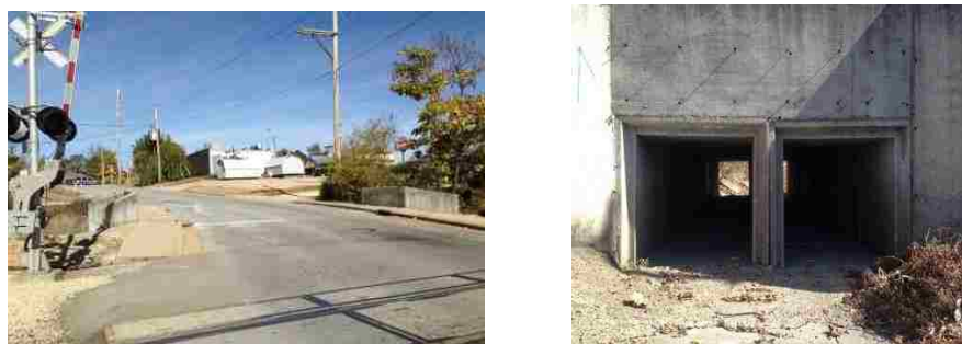
Figure 5.22. The view of new Walker Bridge
