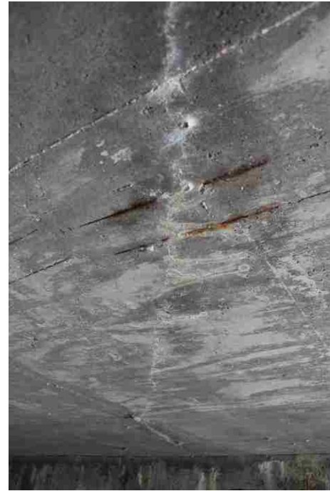
Figure 5.18. The cracks of span 5
