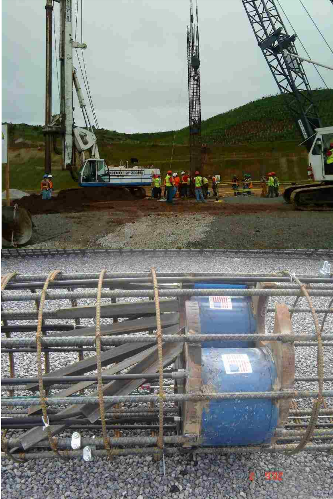
Figure 2.21. Drilled shaft load test of San Juan Cement Plant
