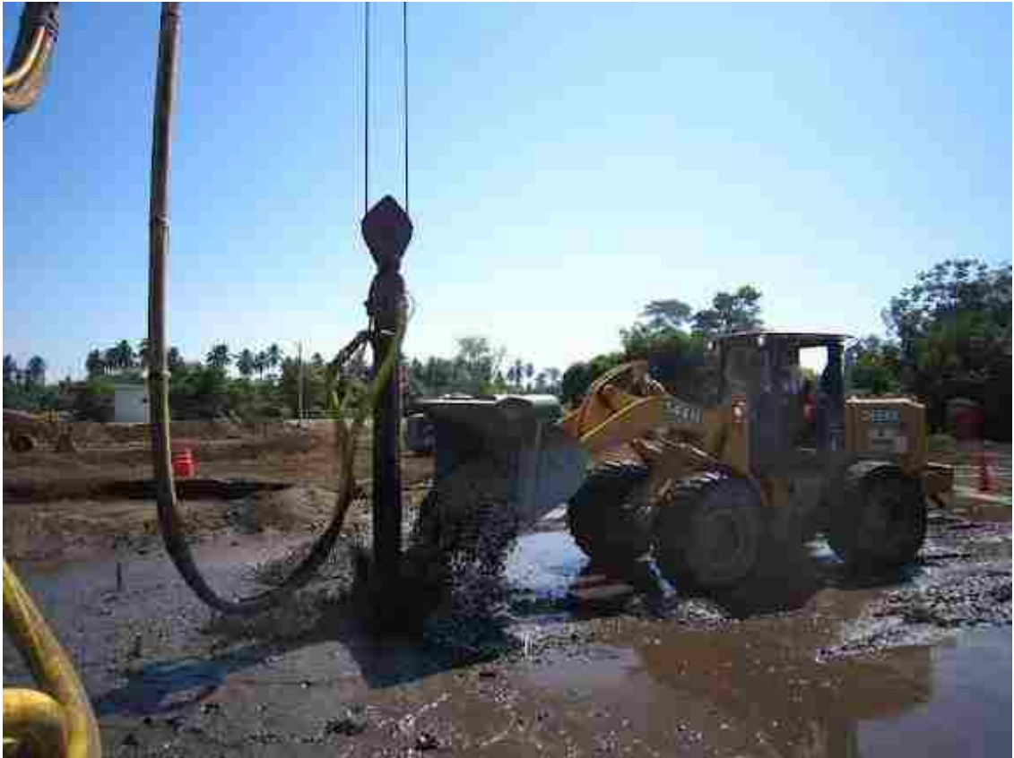
Figure 4.54. Gravel filling and compaction
