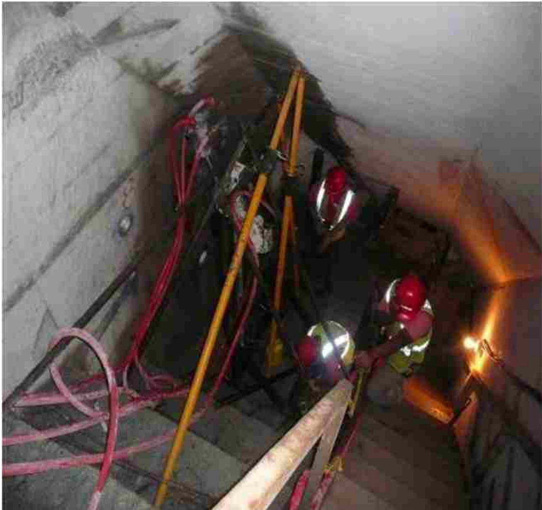
Figure 4.31. Grouting from access gallery using wire line system
