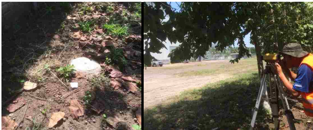
Figure 4.66. Survey monument and surveying works
