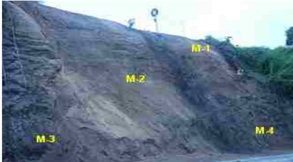
Figure 4.4. Slope face with sampling location
