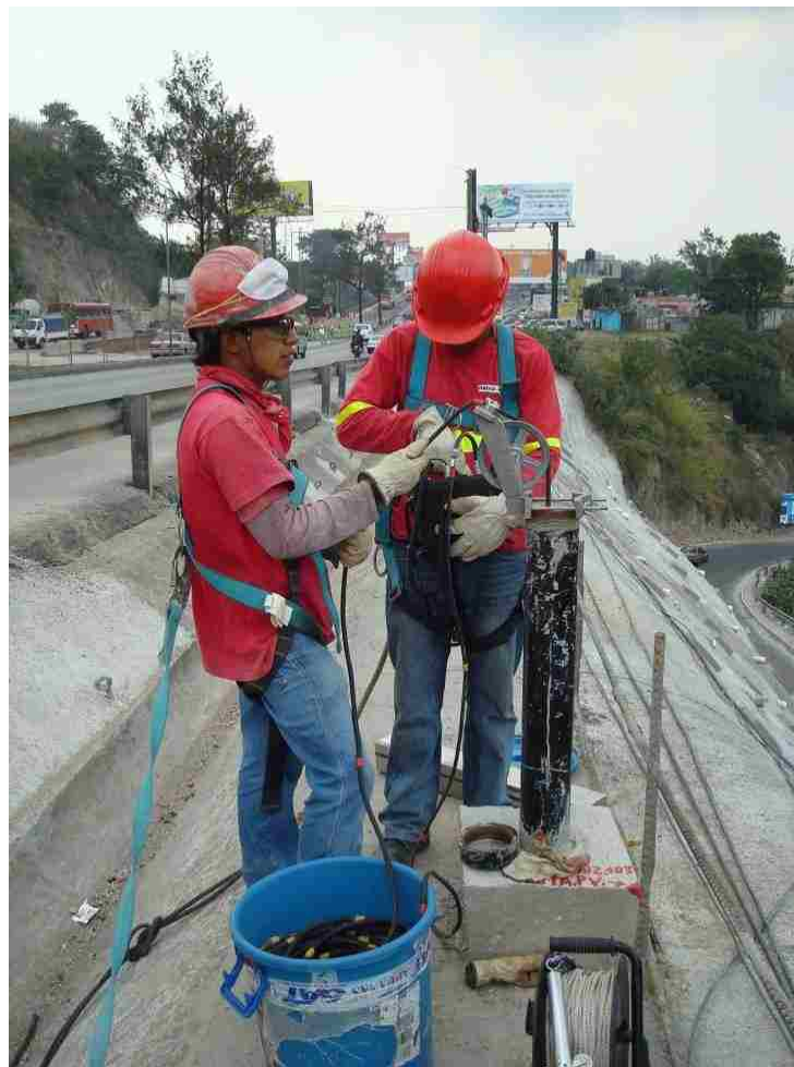
Figure 4.15. Inclinometer reading
