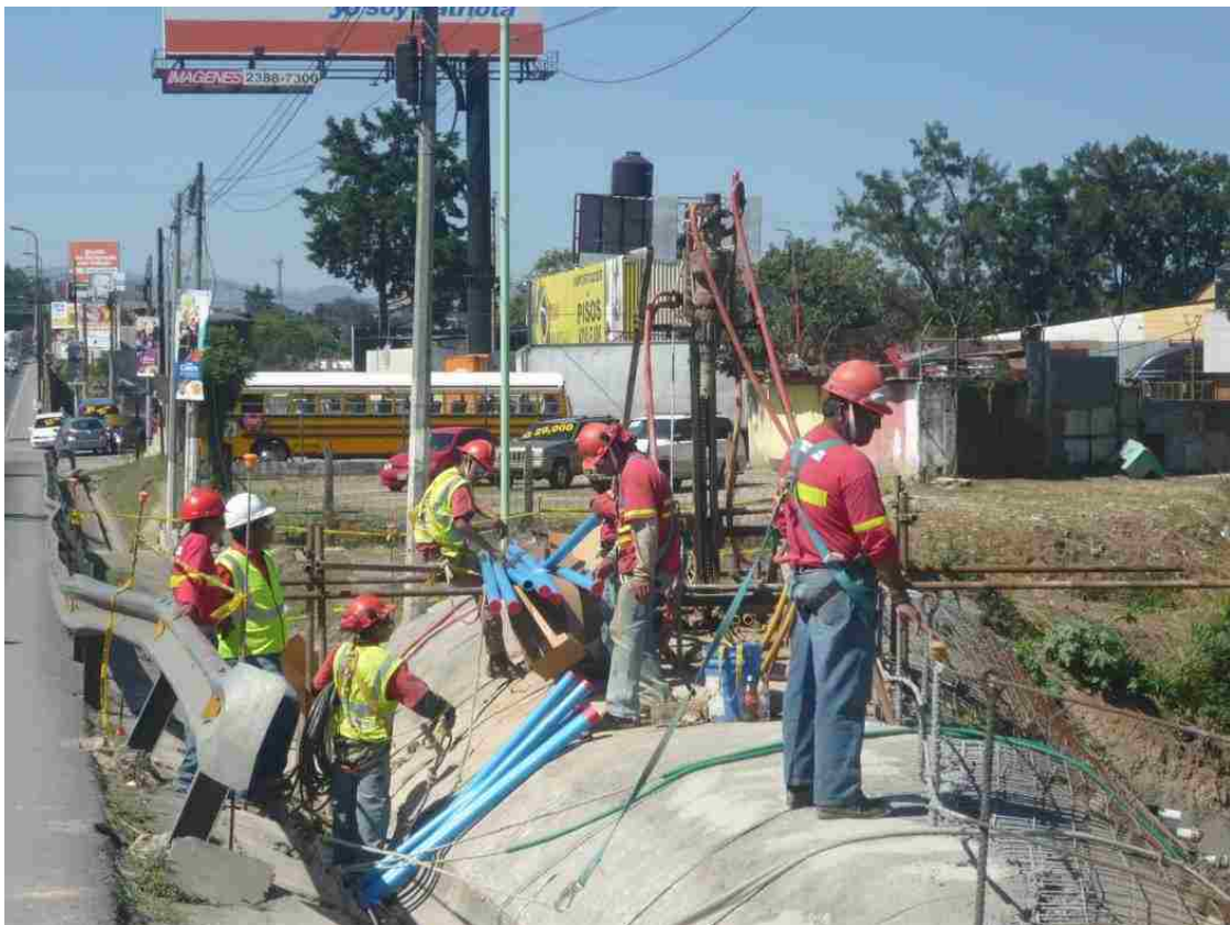
Figure 4.14. Inclinometer installation
