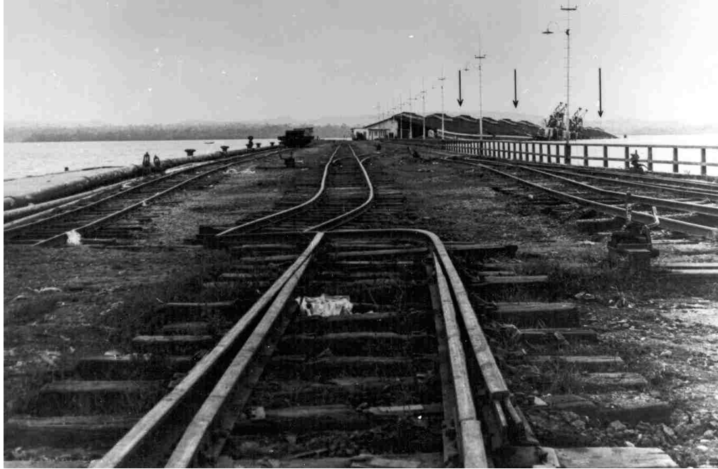
Figure 2.9. Puerto Barrios wharf, destroyed by the February 4 earthquake. Arrows point to the large warehouse partially submerged ((Plafker, 1977)
