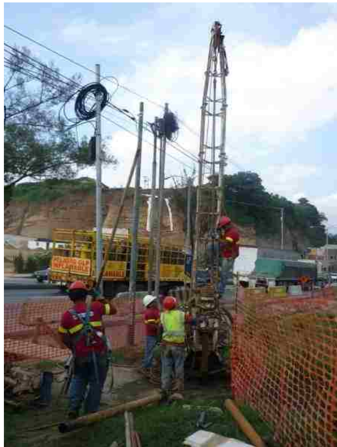
Figure 4.5. Boreholes drilling
