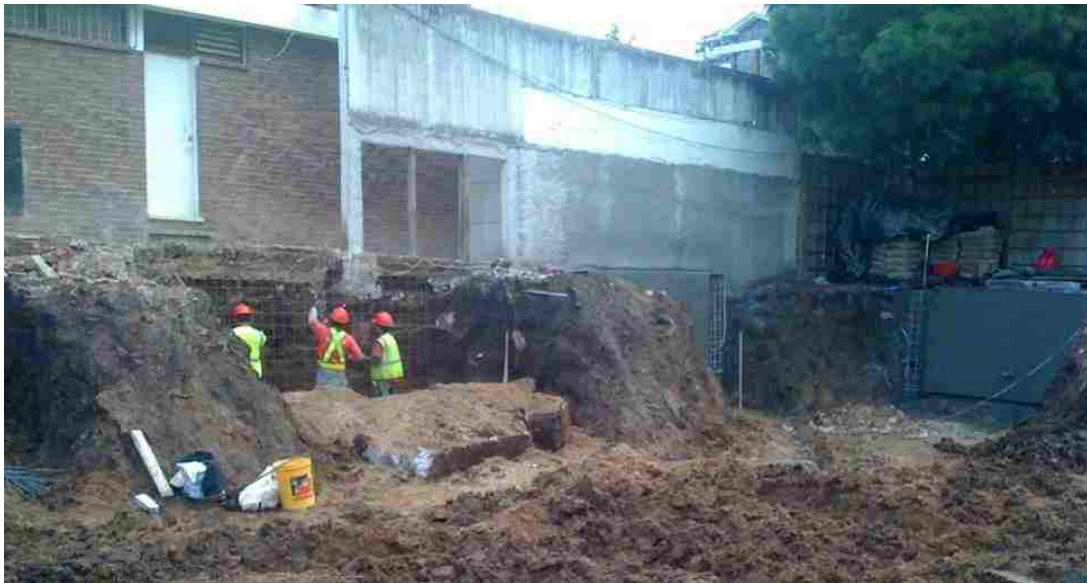
Figure 3.2. Berm utilization during construction
