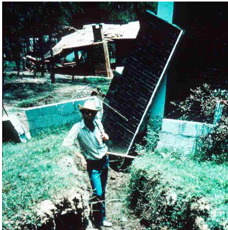
Figure 2.10. Cracks at Lake Amatitlan (Plafker, 1977)
