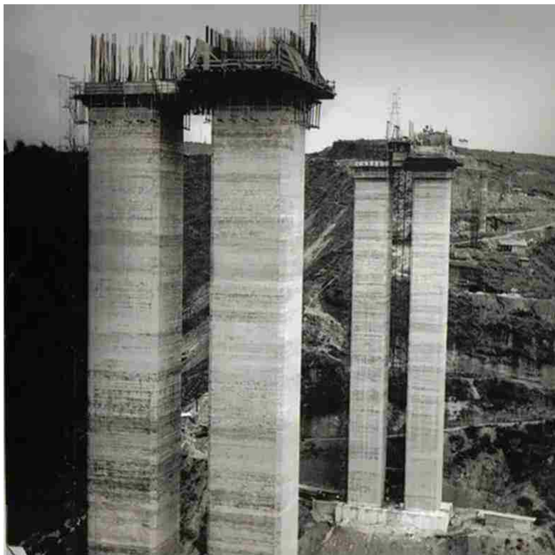
Figure 2.18. Construction of Incienso Bridge piers (Rodas, 2012)
