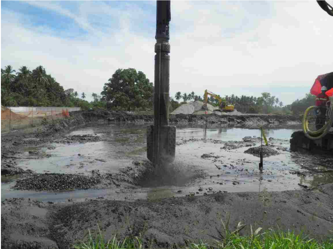
Figure 4.55. Final stage of the compaction process
