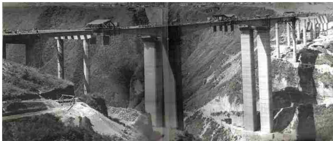
Figure 2.17. Construction of Incienso Bridge deck (Castillo, 2009)
