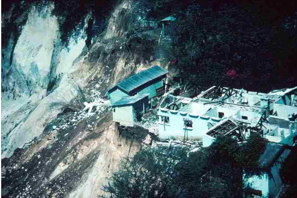
Figure 2.5. Landslide along the edge of a steep walled valley in Guatemala City (Plafker, 1977)
