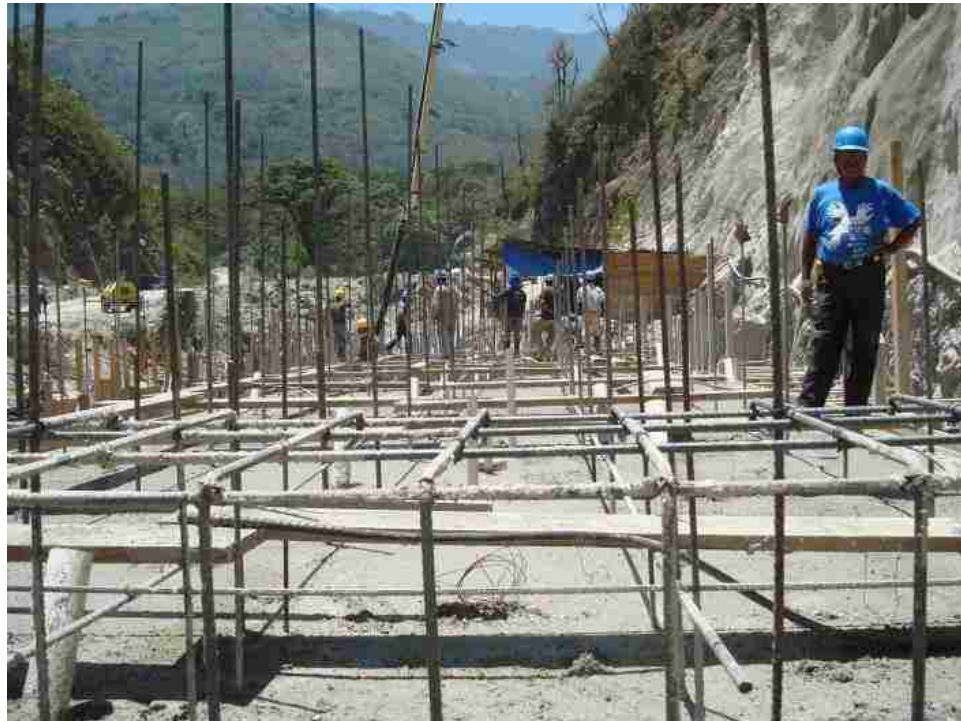
Figure 4.28. PVC sleeves intalled during construction
