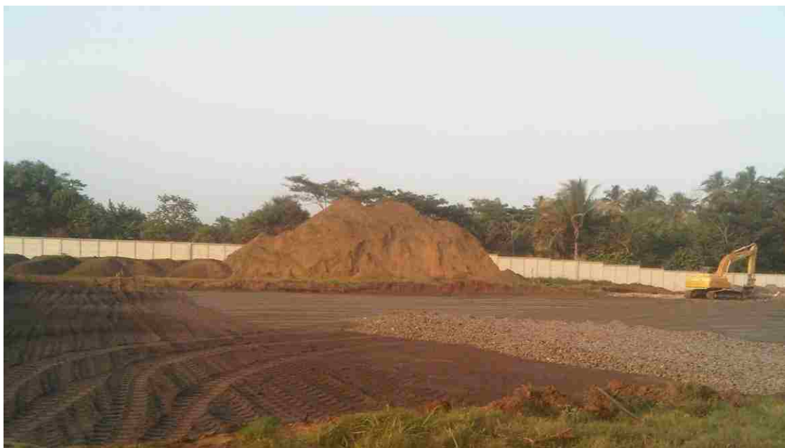
Figure 4.52. Working platform construction
