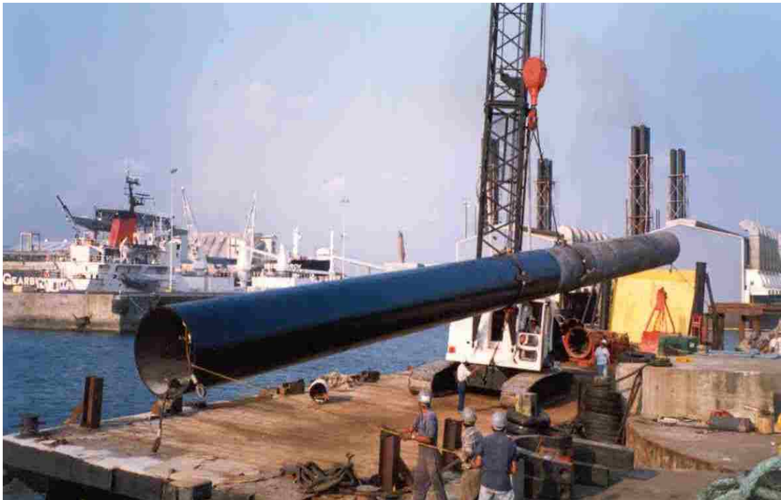
Figure 2.15. Steel piles of Barcaza Man
