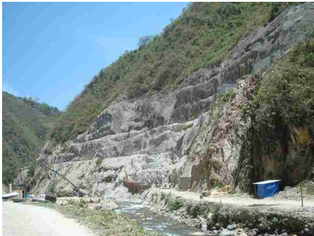
Figure 2.14. Construction site of Santa Teresa Dam
