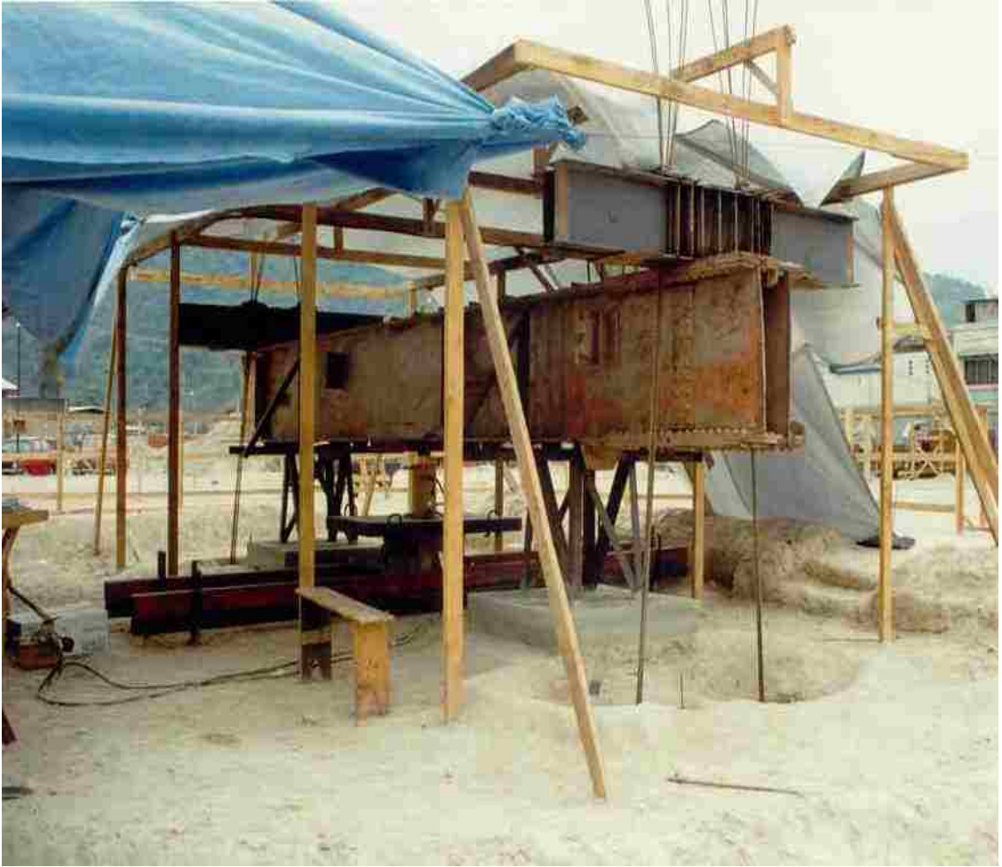
Figure 2.20. Pile load test in Cementos Progreso Cement Plant
