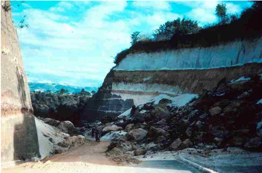
Figure 2.6. Landslides in steep roadcut of stratified pumice and ash deposits at San Cristobal (Plafker, 1977)
