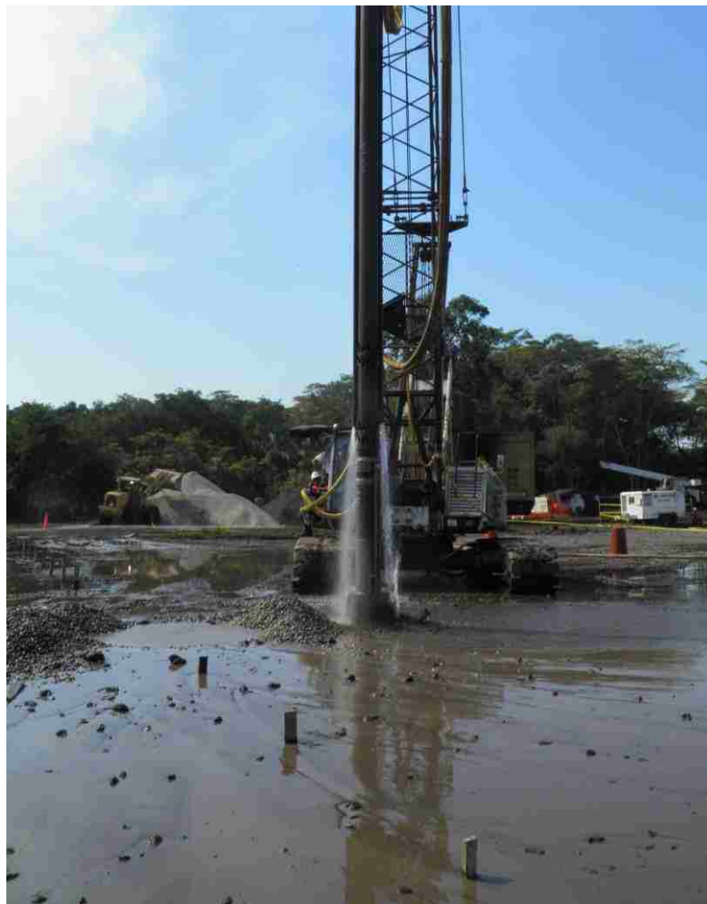
Figure 4.53. Vibroflot penetration
