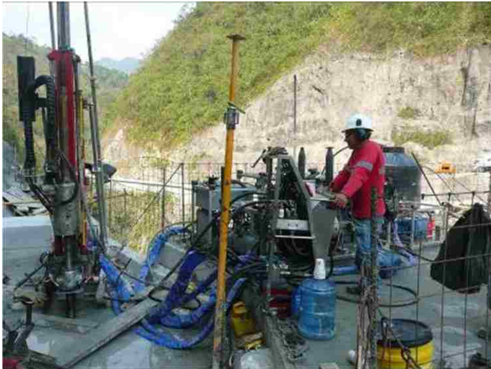
Figure 4.30. Drilling from the surface using wire line system
