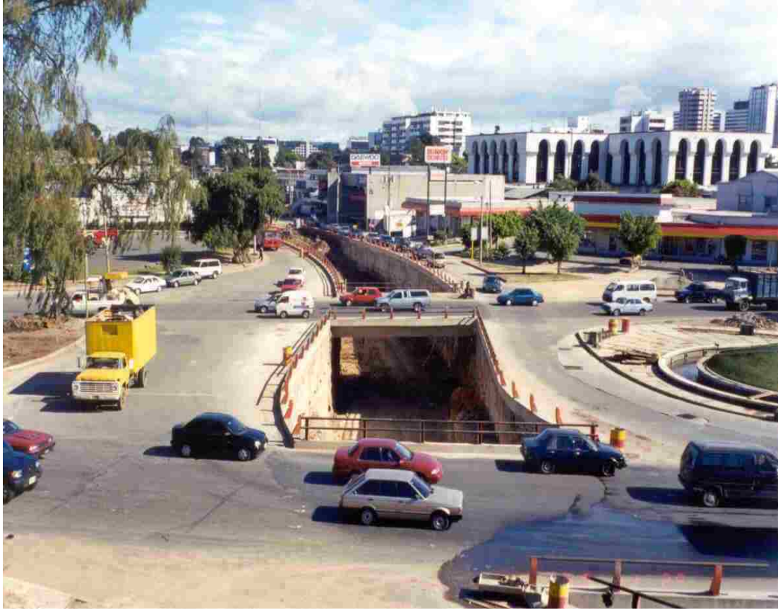
Figure 2.19. Construction of Reloj de Flores Underpass
