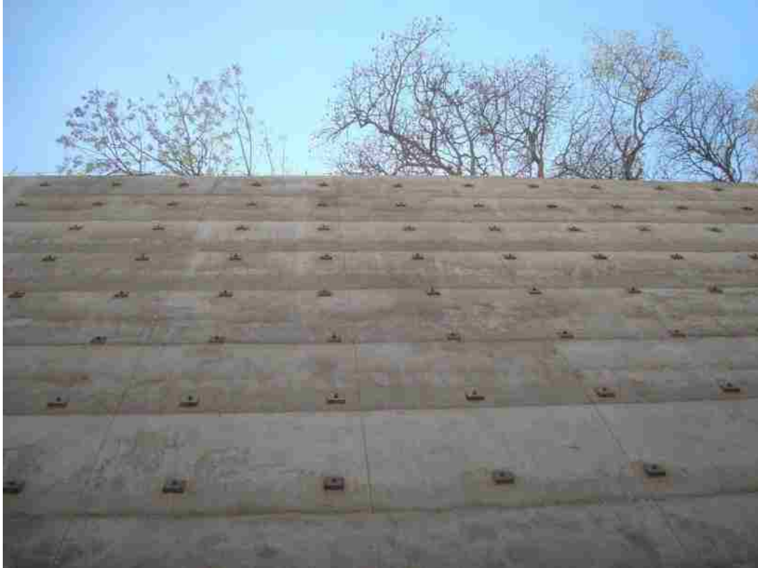
Figure 3.1. Vertical soil nailing wall for excavation stabilization
