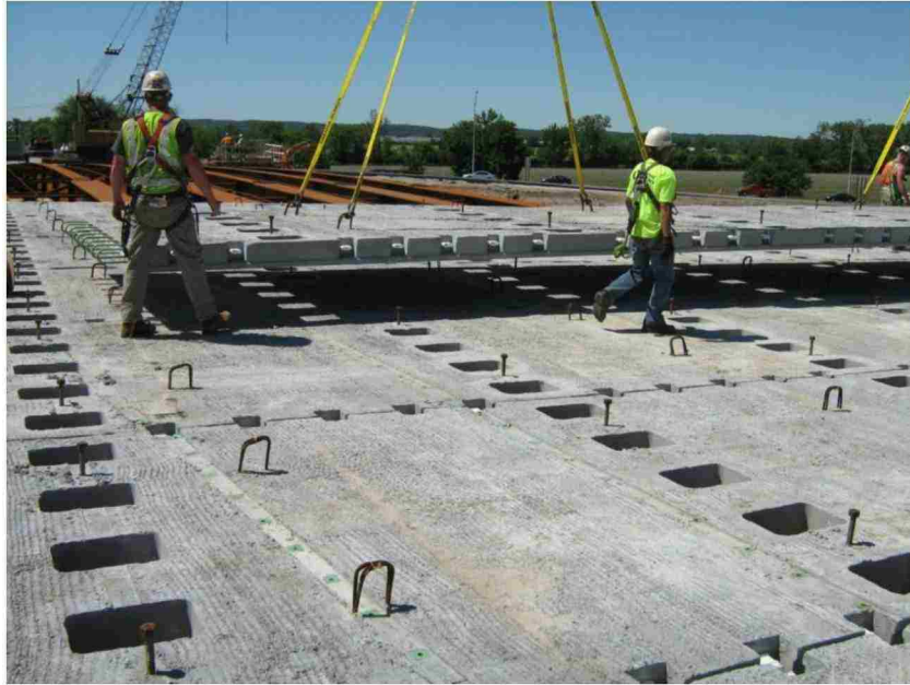
Figure 2.5. Bridge deck being constructed with full-depth precast concrete deck panels (Chavel, 2012)
