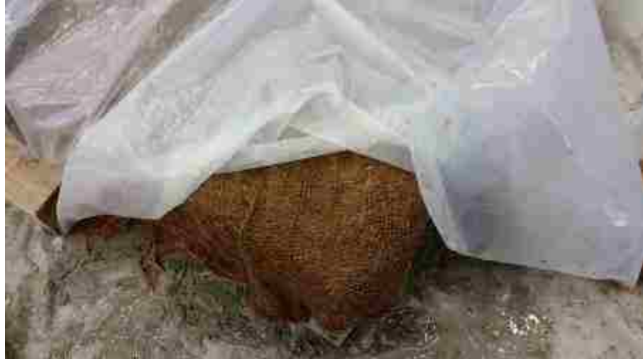
Figure 5.10. Wet burlap on top of concrete surface
