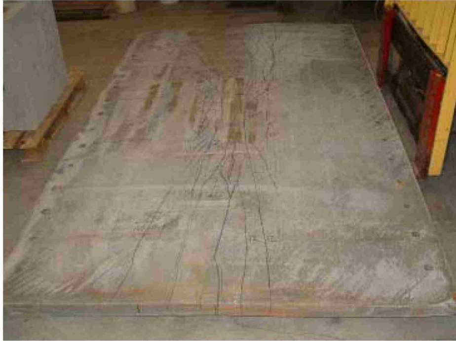
Figure 2.12. Typical cracking pattern on bottom surface of the panels (Harris & Roberts-Wollmann, 2008)
