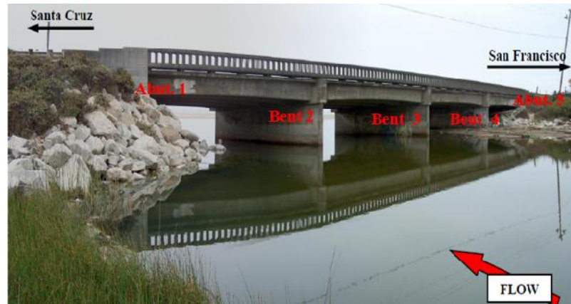
Figure 5.12. State Highway 1 Bridge over Waddell Creek, CA.
