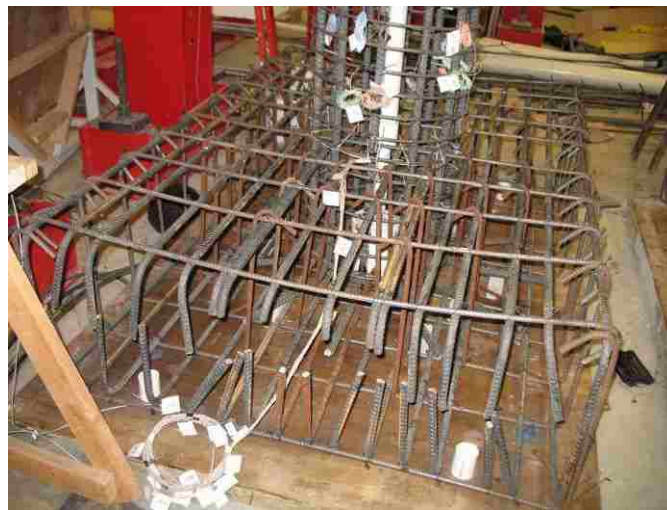
Figure 3.15 Finished Foundation Reinforcement with Column Cage
