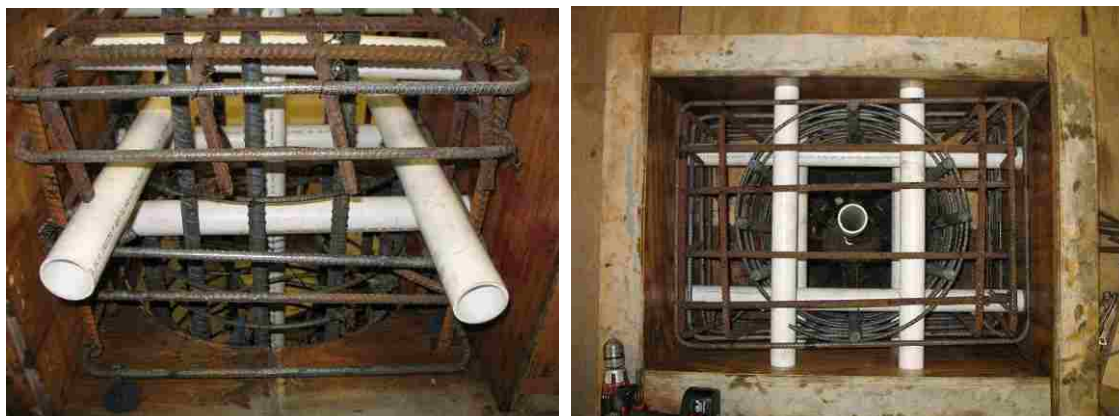
Figure 3.16 Formwork and PVC Layout on Loading Block
