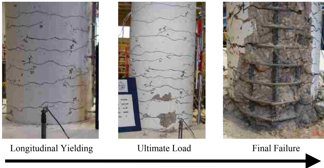
Figure 4.4 Damage to Column H/D(6)-T/M (0.0)-0.73% under Flexure
