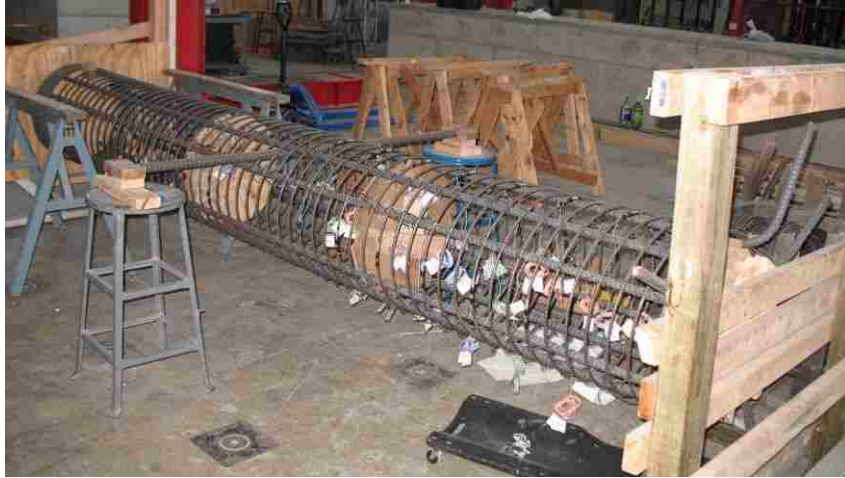
Figure 3.13 Fabrication of Column Cage
