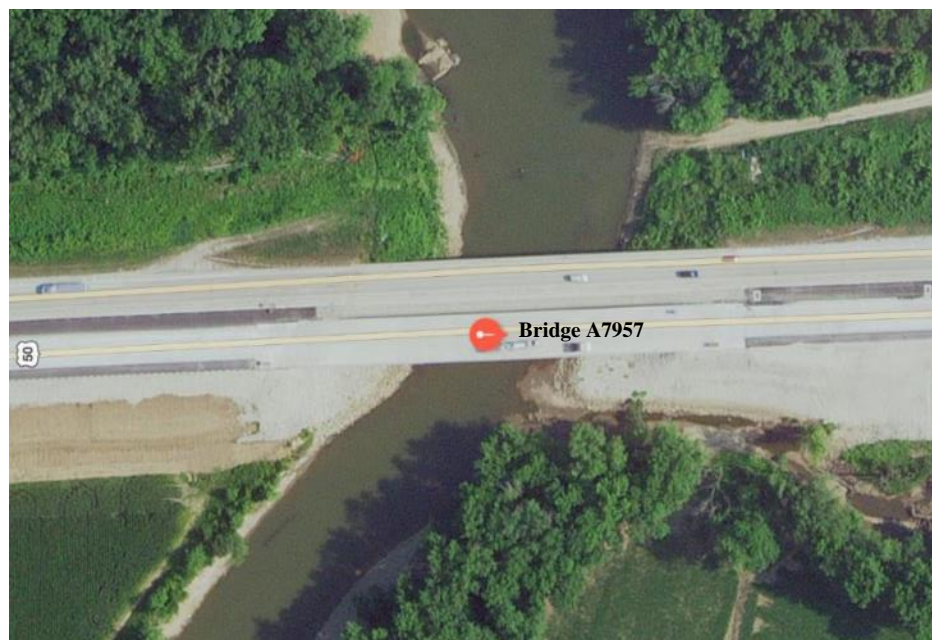
Figure 1.10. Aerial View of the A7957 Bridge
