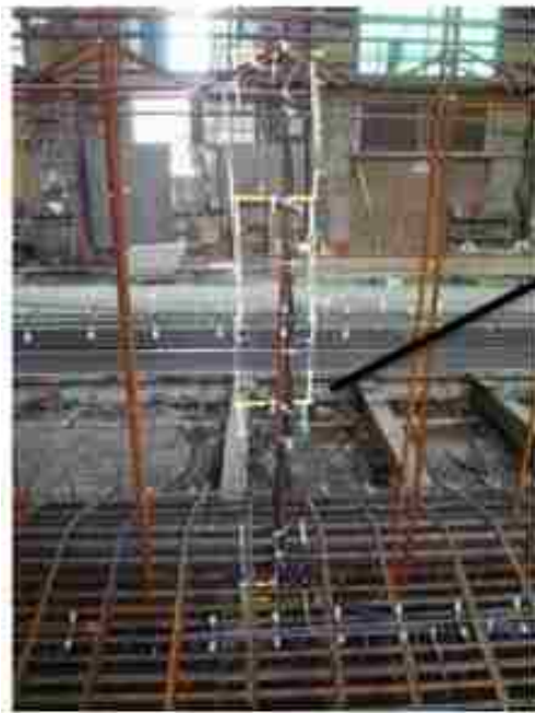
a) VWSGs in the midspan
