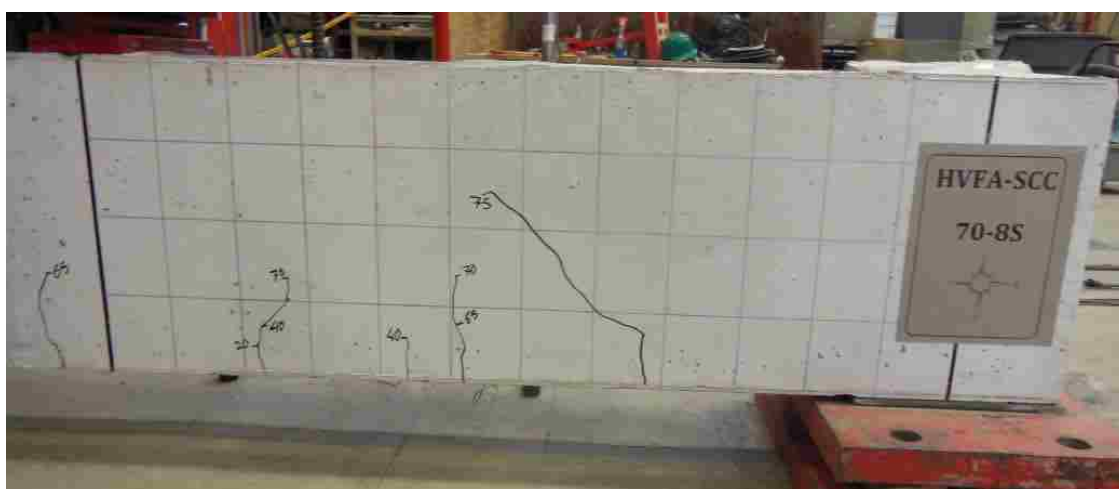
Figure B-22. Cracking Shear in Specimen 70-8S
