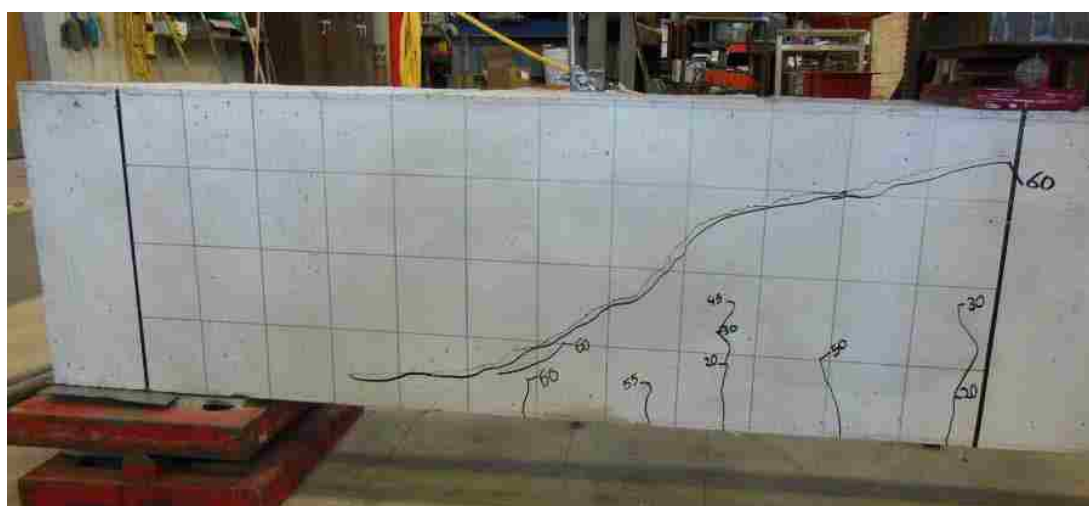
Figure B-18. Cracking Shear in Specimen 70-6N
