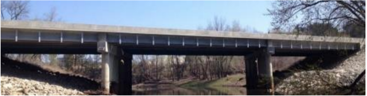
Figure 2. Bridge A7957 during the summer.
