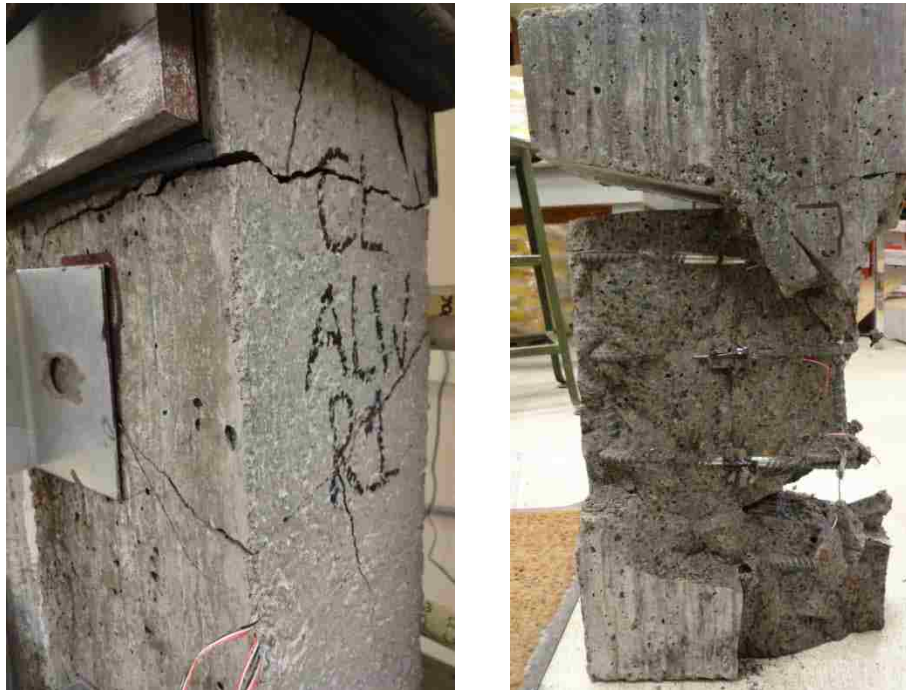
Figure 3.61 Concrete Cracking on A-CL-CJ-R-1 (left), After the Removal of All Loose Concrete (right)
