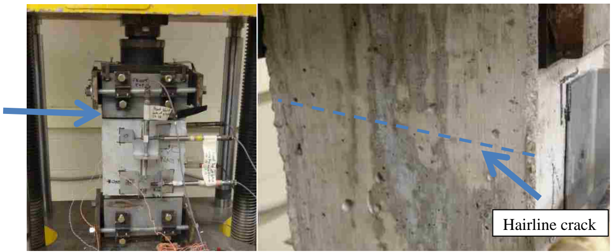
Figure 3.20 Location and Example of Hairline Flexural Cracks
