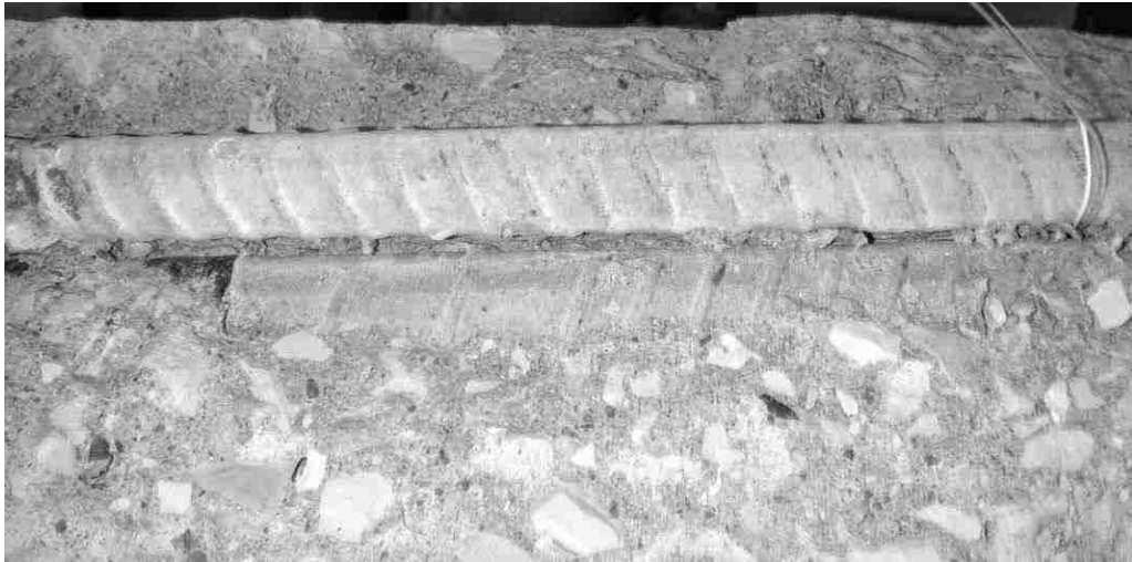
Figure 5.3. View of Enamel Coated Rebar in Splice Region of Beam 6C32N
