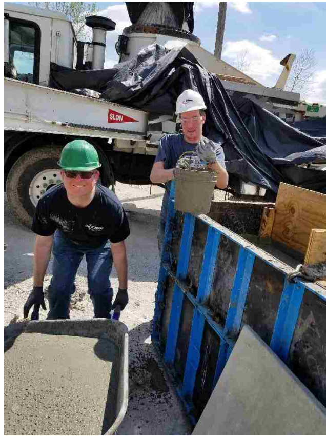
Figure 4-9 Concrete transportation using a wheel barrow.
