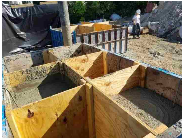
Figure 4-8 Formwork used to discharge pumped concrete.
