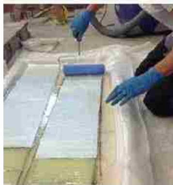
Saturate fiber in epoxy
