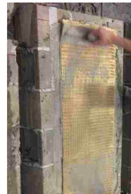
Apply fiber on matrix
