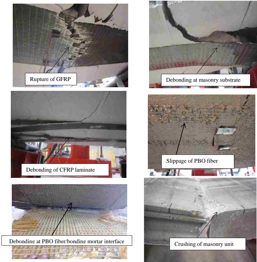
Figure 6. Typical mode of failures
