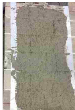
Apply matrix on wall
