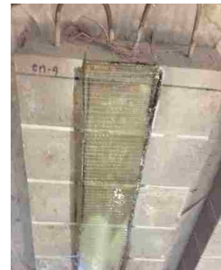
Apply saturated sheet on wall
