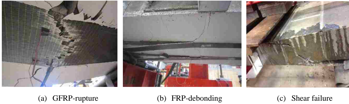
Figure 7. Observed modes of failure
